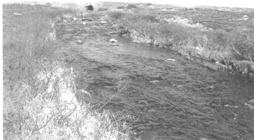
Figure-7 Confined gravel ditch for effluent to Bake Lake
