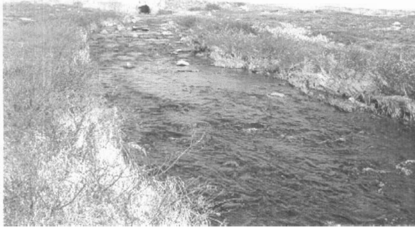
Figure-5 Confined gravel ditch for effluent to Baker Lake
