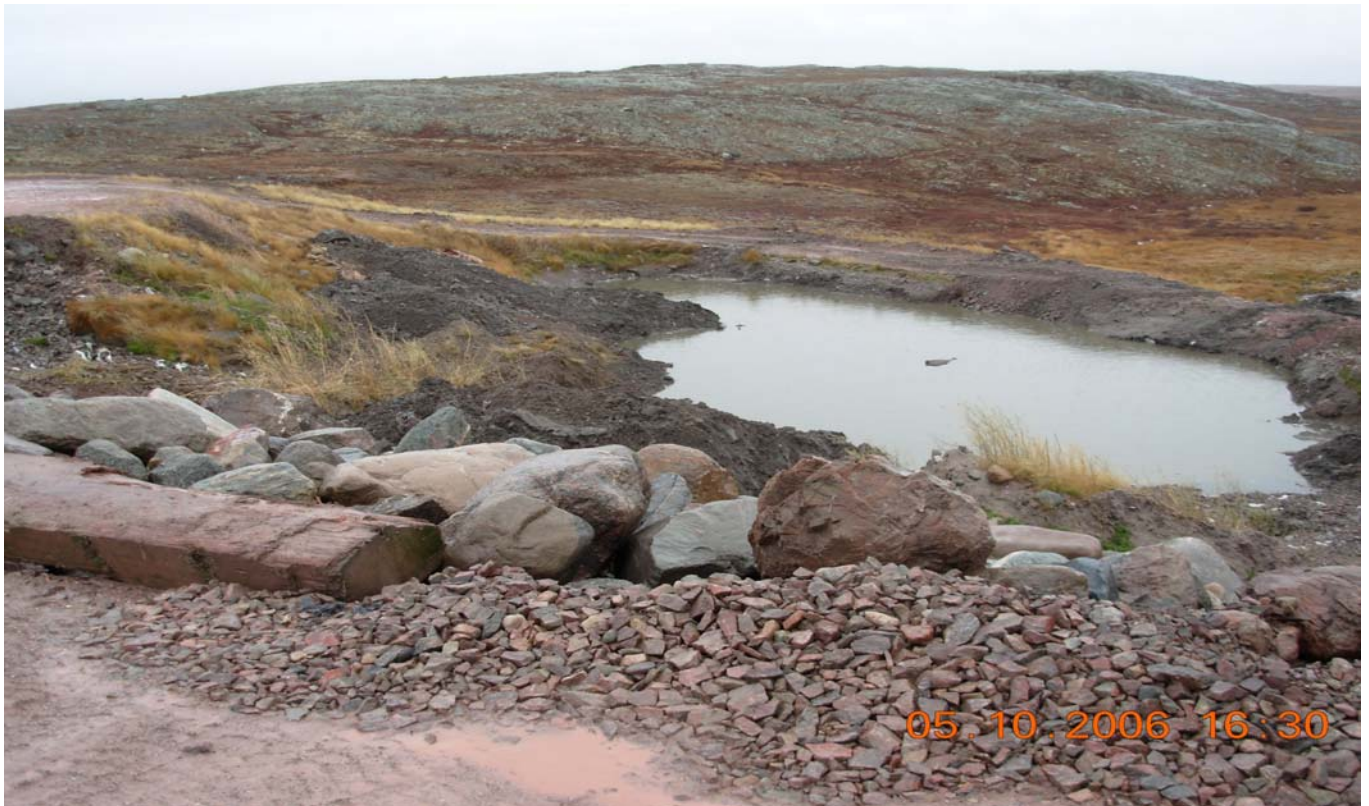
Photo 2 - Holding Cell in October 2006, after berm repaired, discharge by exfiltration.
