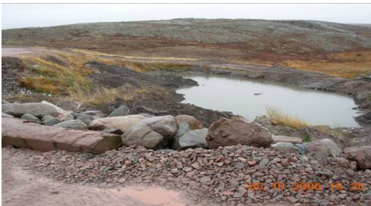
Photo 2 Holding Cell in October 2006, after berm repaired, discharged by exfiltration.
