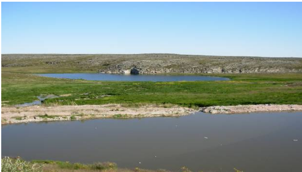
Photo 1 Holding Cell (foreground) looking to Lagoon Lake, main discharge is through breach in berm (August 2006).
