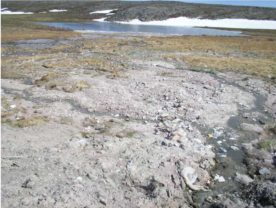
Figure 5: Water leaking out of the base of the berm flowing through two channels towards Lagoon Lake.
