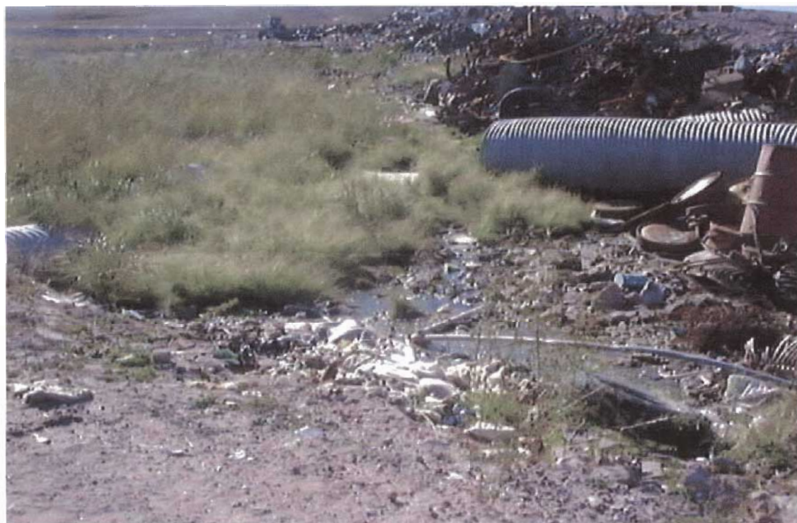
figure 3. Pooled water along the toe of the solid waste disposal facility; 2001/08/31.
