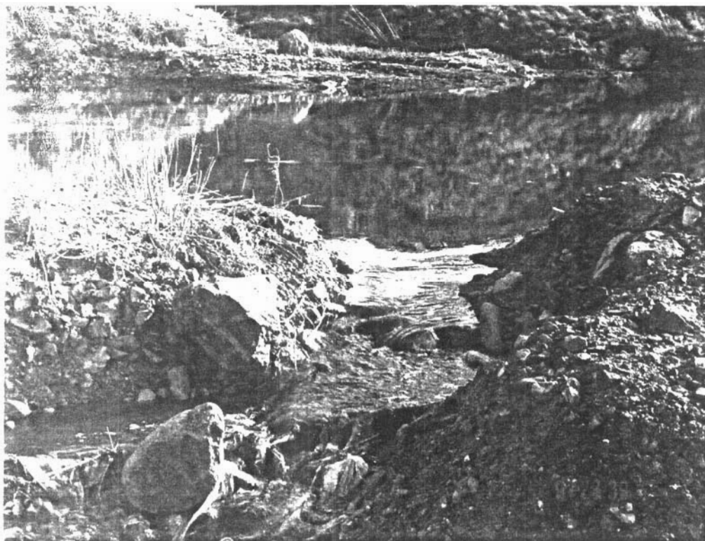
Photo # 6. Sewage effluent exiting lagoon within seconds of truck discharge into sewage lagoon.
