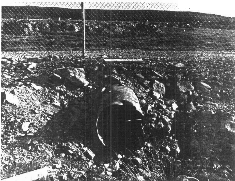
Photo # 12. One of 3 culverts that drain seepage from Solid Waste Disposal Facility,
