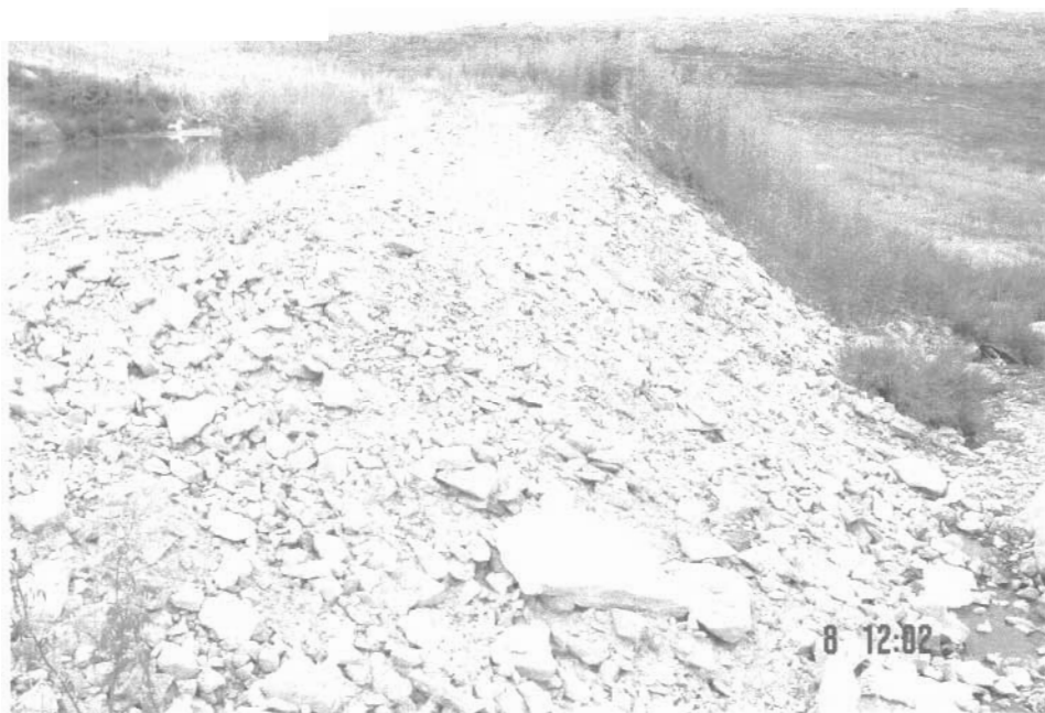
Figure 4. Washed out and replaced section of Hamlet of Baker Lake sewage lagoon.
