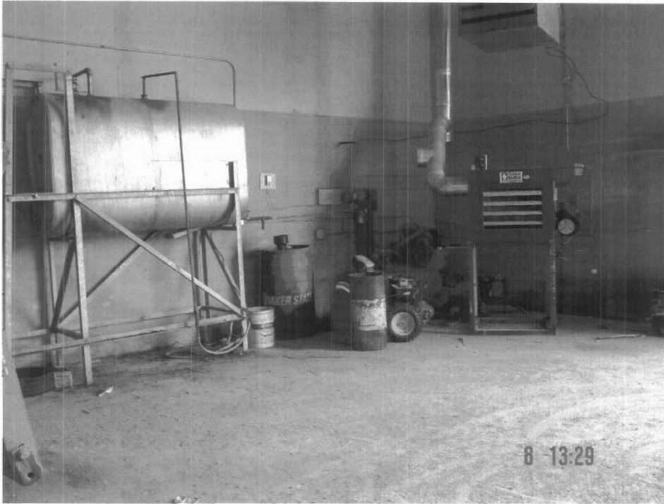
Figure 7. Waste oil container and burner in warehouse in the Hamlet of Baker Lake.
