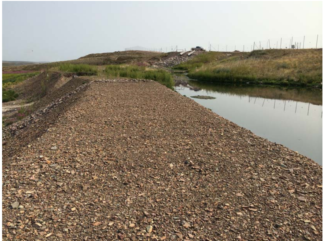
July 29, 2014 – breach in sewage holding cell berm
