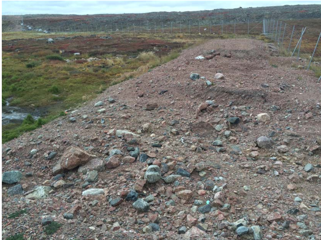
July 29, 2014 – breach in sewage diversion berm
