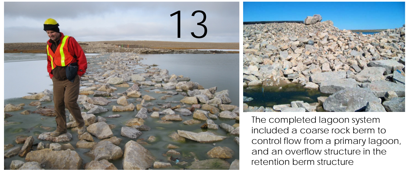
The lagoon is discharged seasonally by pumping over the berm structure through the wetland and onto a slope that cascades into the ocean in a location further away from the community - the measured effluent quality is BOD 25 to 50 mg/L; TSS 50 to 100 mg/L and FC 400 to 4000 CFU / 100 mL
