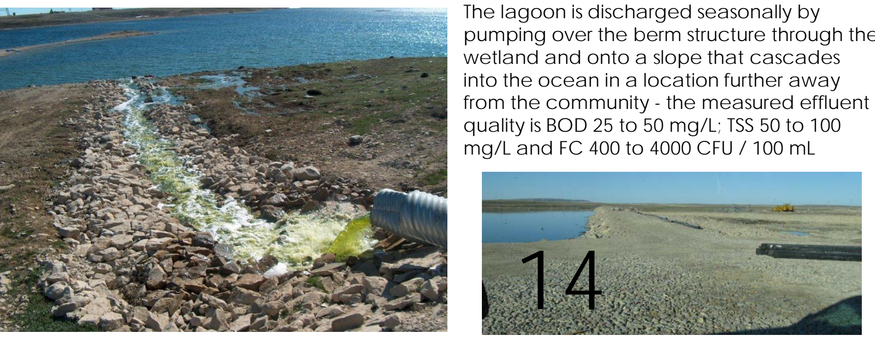
The completed lagoon system included a coarse rock berm to control flow from a primary lagoon, and an overflow structure in the retention berm structure
