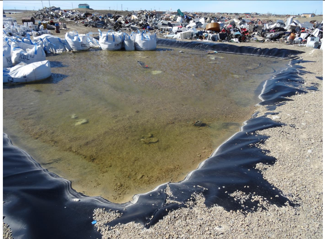
Description: Berm #2 within the Metal Dump showing Melt Water and Mega Bags requiring removal/relocation
