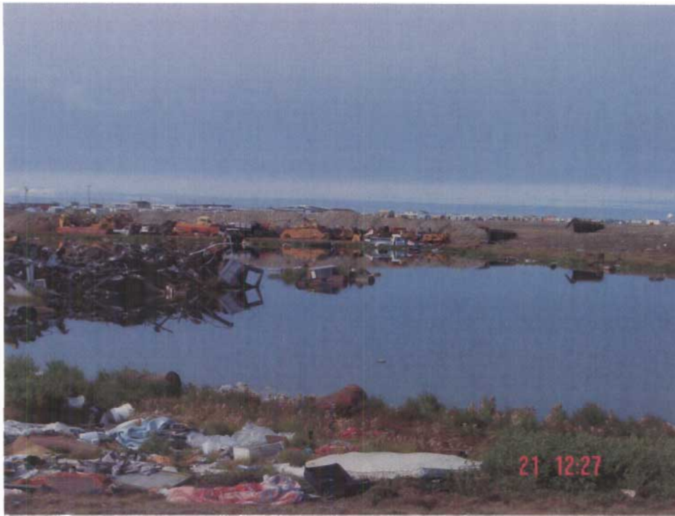
Photo # 5 Bulky metal waste containment area. Note that there is sewage effluent flowing through bulky metal materials.
