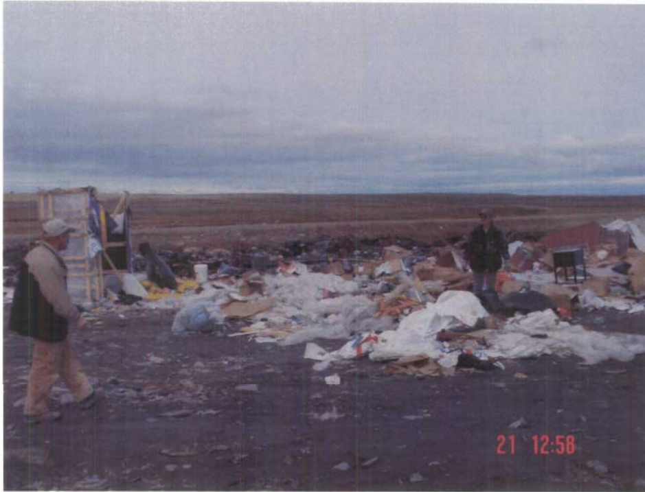
Photo # 7 Tipping face at Solid Waste Disposal Facility. Note burning of refuse occurs on a frequent basis reducing wind blown refuse despite lack of fencing.
