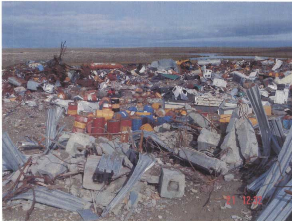
Photo # 7 Tipping face at Solid Waste Disposal Facility. Note burning of refuse occurs on a frequent basis reducing wind blown refuse despite lack of fencing.
