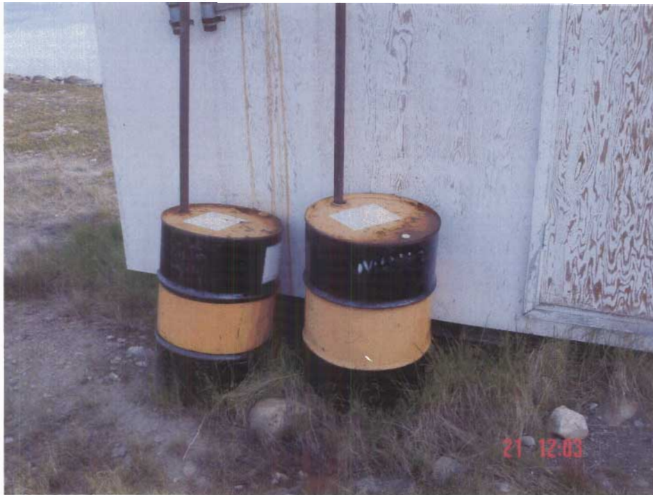
Photo # 3 Over flow for fuel oil at Water Intake Facility, staining of fuel noted around drums.
