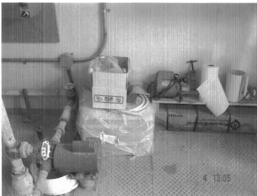
Photo 3. Chlorination system at Water Intake Facility.
