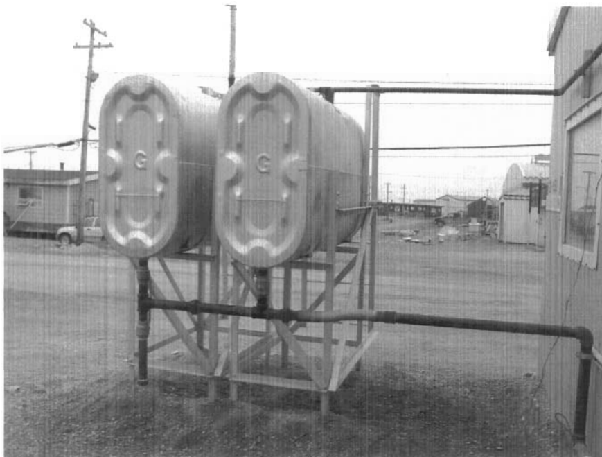
Photo 13. Fuel tanks at Water Treatment Plant require a berm.
