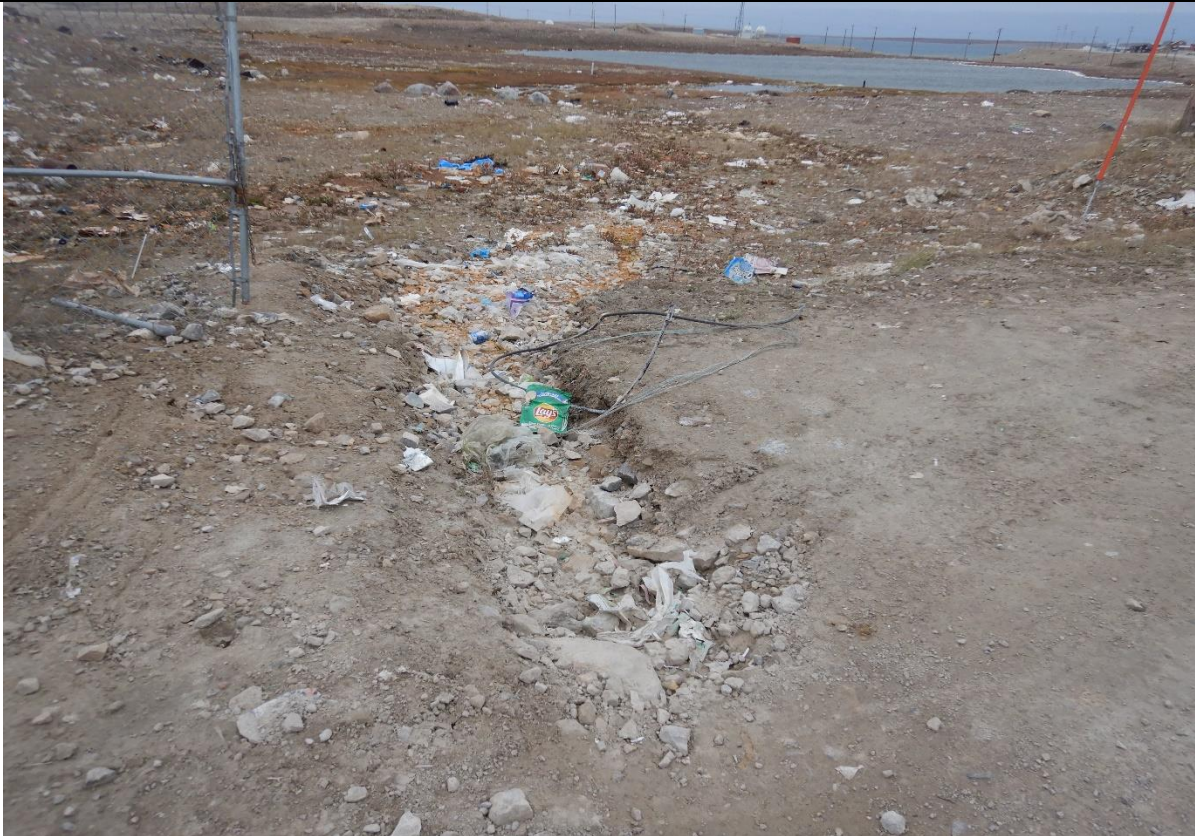
Description: erosion near landfill entrance indicating effluent leaving the facility
