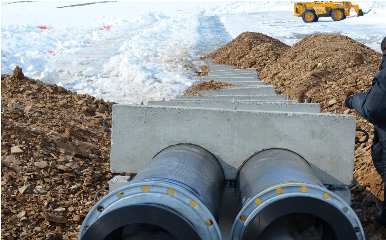
HDPE buried line from new IPH to vault #16
