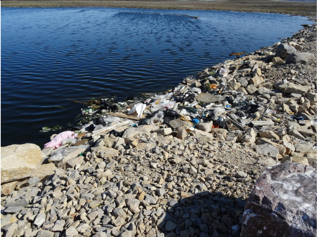
Description: The Sewage Lagoon Berm Run-off area showing less than 1 meter Free Board
