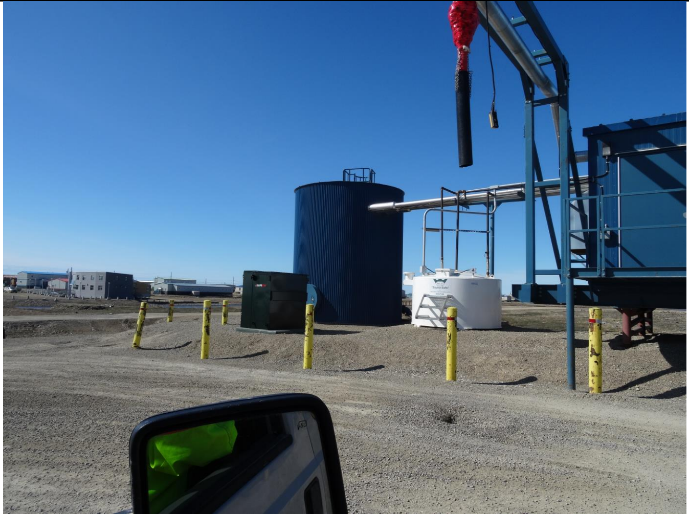
Description: The Back Wash Tank attached to the Water Plant
