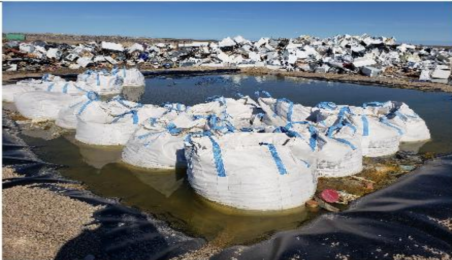
Description: second cell with room for Hazardous material containment
