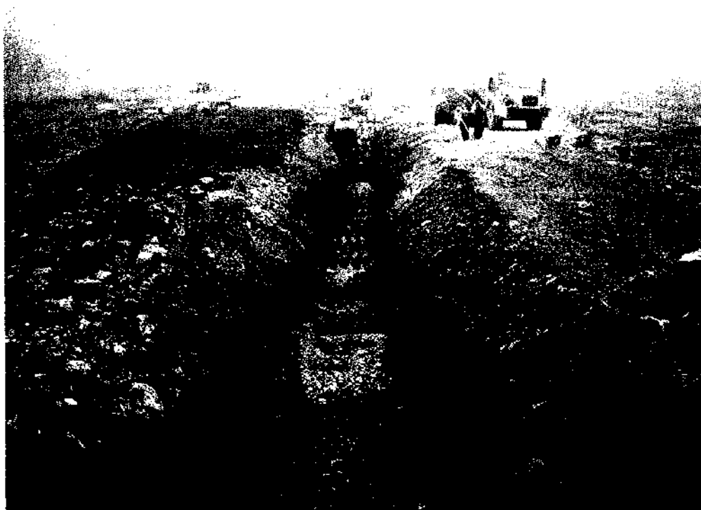
Photo 2: Excavating cut off trench 2 in clay, station 190m to 150m
