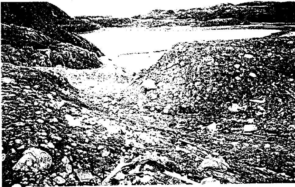
Photo No. 7: Cape Dorset Landfill - View North West of Breached Berm
