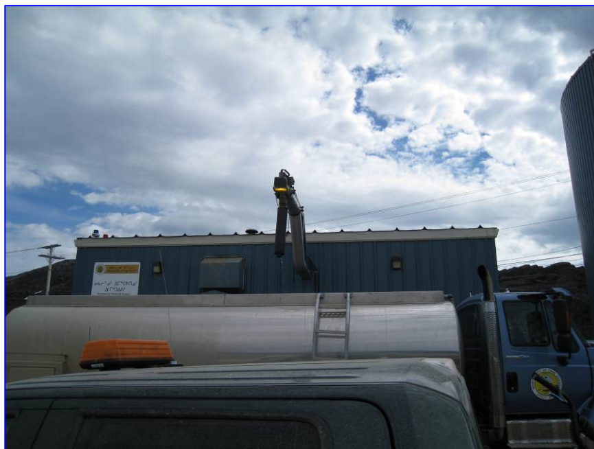
Photograph No. 14 Truck fill station
