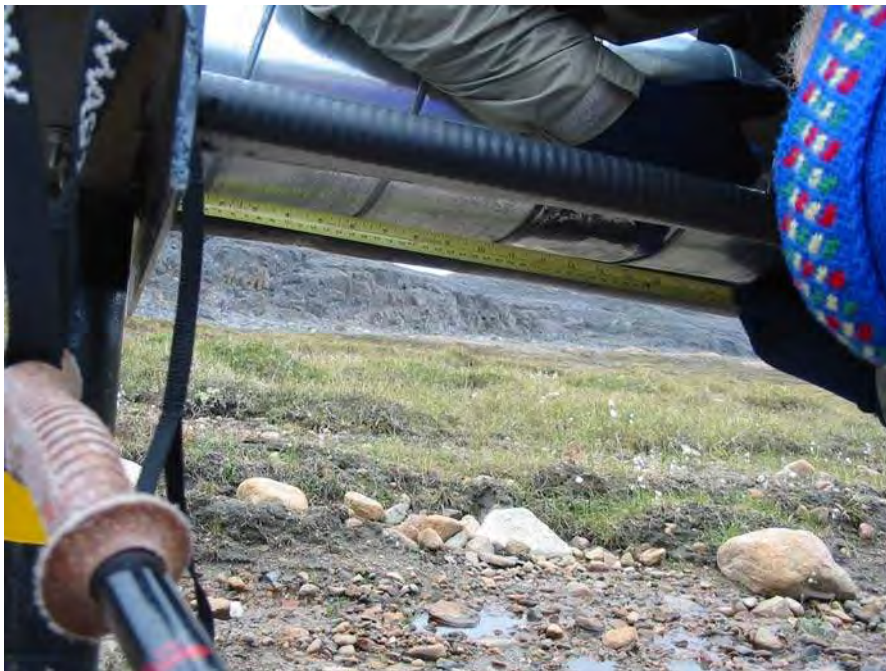
Photograph 22: Approximately 310 metres below of expansion loop, displacement of approximately 15 inches.
