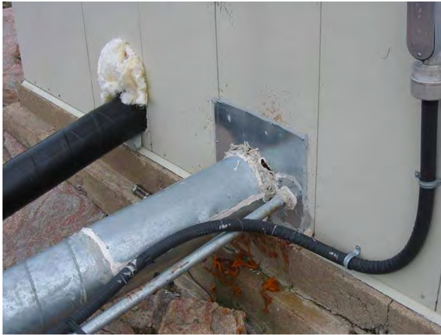
Photograph 5: Pipe penetration through the wall of the Heater House, the condition of the caulking demonstrates piping movement.
