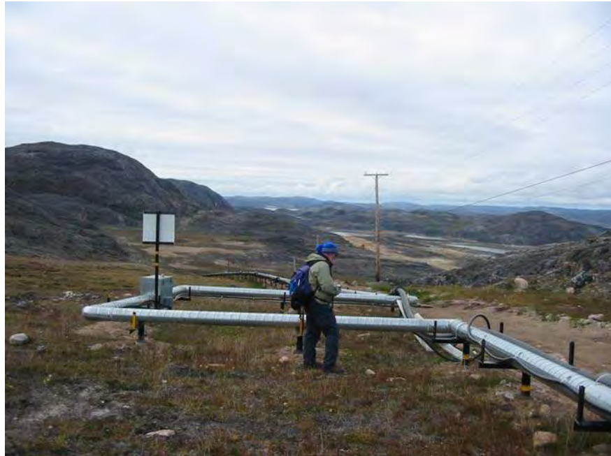
Photograph 15: The uphill leg of the expansion loop illustrates a lateral displacement of approximately two inches at the two pipe supports. (See photograph 16)
