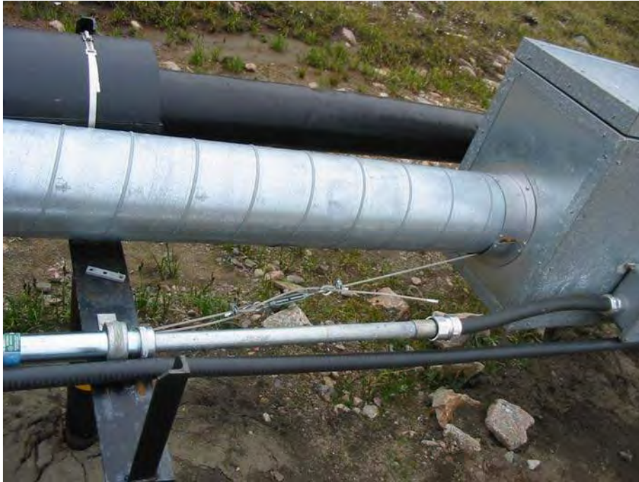
Photograph 21: Approximately 265 metres downhill of expansion loop. A temporary cable restrain that has been installed into the junction box by the Hamlet.
