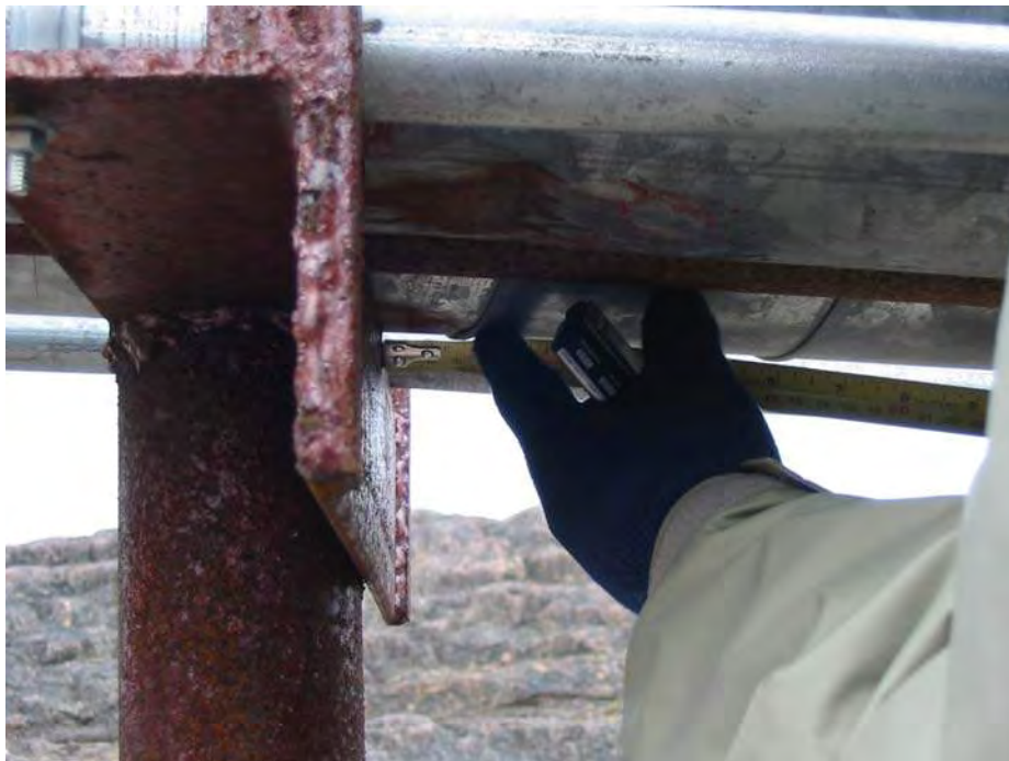
Photograph 4: Downhill of the Heater House towards Tee Lake. The photograph illustrates a displacement of 1.25 inches.
