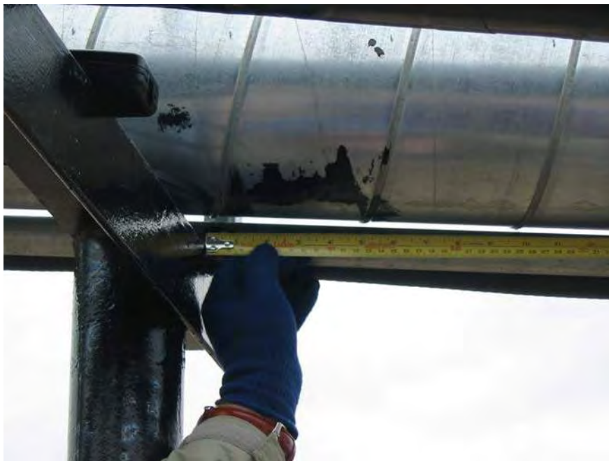
Photograph 30: Approximately 65 metres downhill of road crossing displacement of approximately 5 inches down slope.
