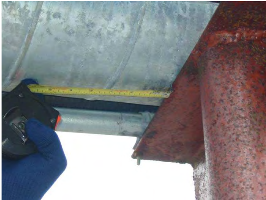
Photograph 10: At the elevated section of the pipe. Photograph illustrating a displacement of approximately one inch.
