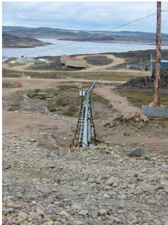
Photograph 28: Photograph is taken from the road looking down the pipeline. Note that the pipeline is straight to the next junction box but has some observable displacements beyond the junction box.
