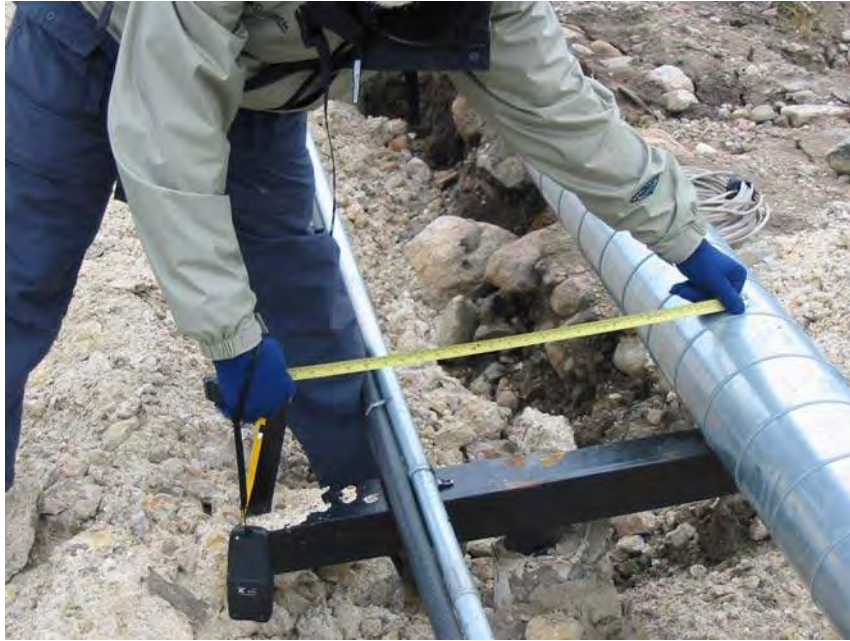
Photograph 27: Pipe has displaced laterally approximately 13 inches on the supports above the road crossing.
