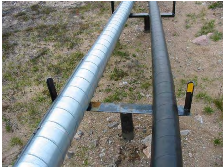
Photograph 14: The pipeline is displaced off centre on the pipe support. Paint marks indicate little movement.
