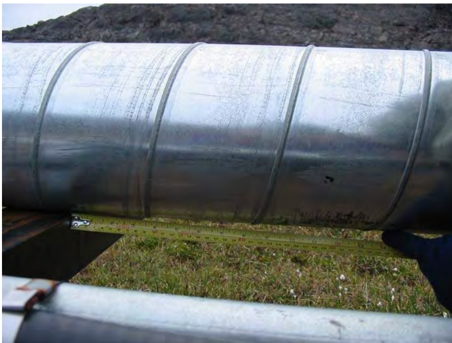
Photograph 18: Displacement downhill of the pipeline by approximately 14.5 inches at approximately 20 metres below the expansion loop.
