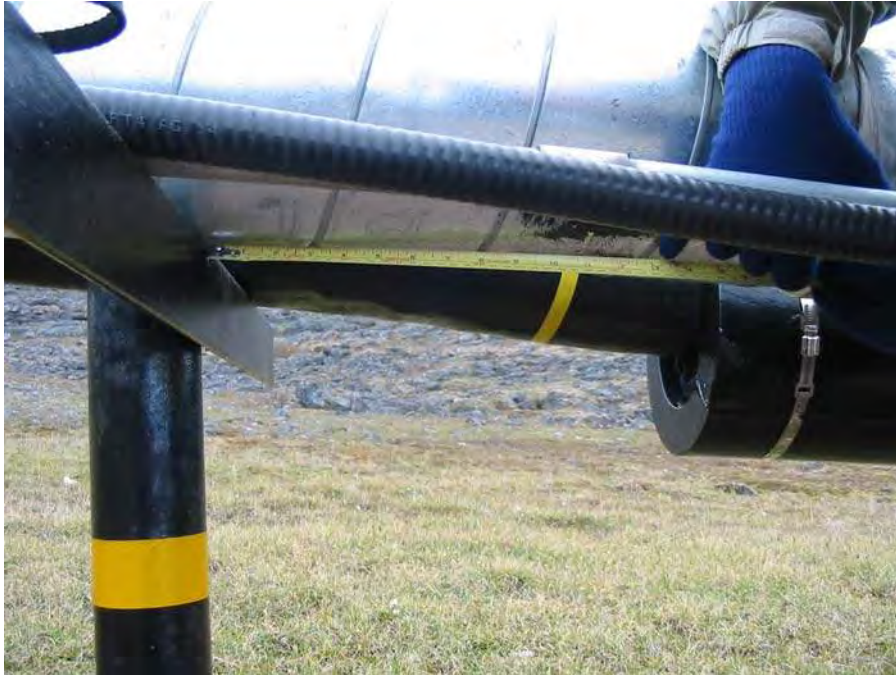
Photograph 19: Approximately 180 metres downhill of expansion loop, displacement of approximately 14 inches.
