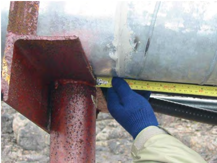
Photograph 8: Elevated section of pipeline immediately above where the road crosses underneath the pipeline. The photograph illustrates a displacement of approximately one inch.
