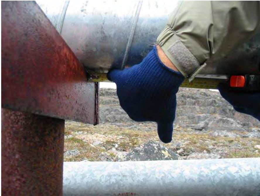
Photograph 3: Immediately below the junction box, between the Heater House and Tee Lake. Photograph illustrates a displacement of approximately 1.5 inches.
