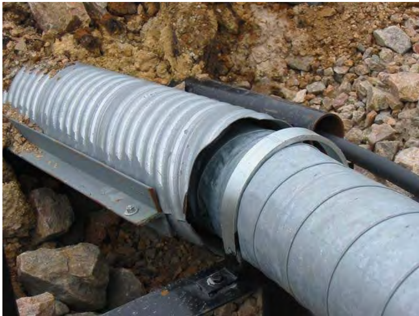
Photograph 26: Bend due to buckling uphill of road crossing.
