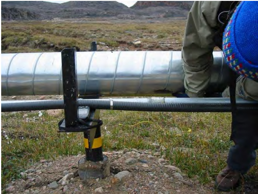
Photograph 23: Approximately 60 metres above the road crossing, displacement of approximately 14 inches.
