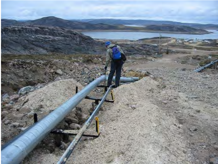
Photograph 25: At the road crossing. The pipe downstream from the bend was originally installed in a straight line but has buckled laterally approximately 20 inches.
