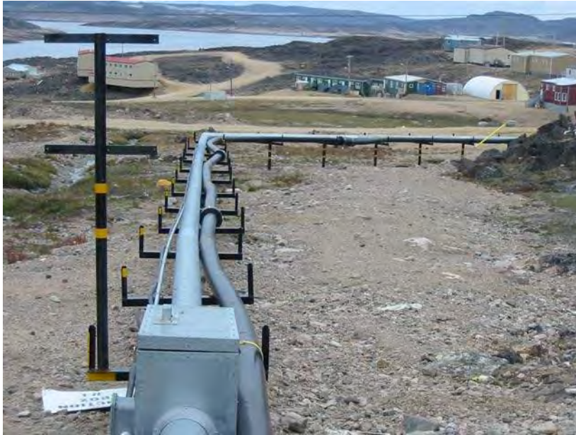
Photograph 31: Photograph depicts the lateral displacement of the pipeline below junction box no. 2.
