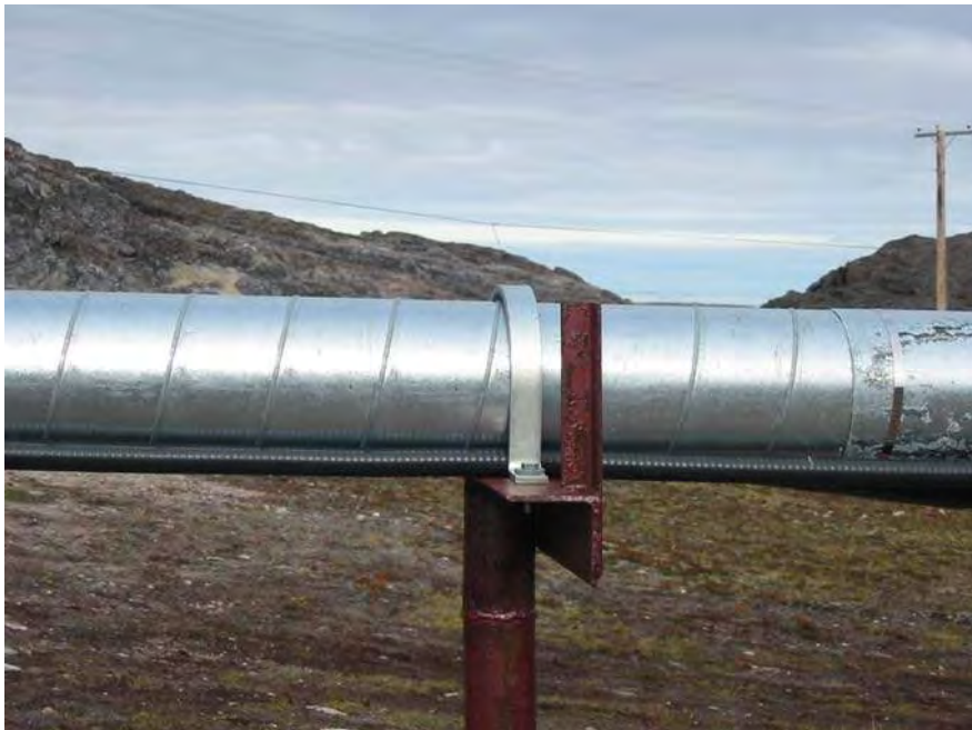
Photograph 12: Photograph of one of the straps over the pipe. The strap is larger in diameter than the outside diameter of the pipe jacket.
