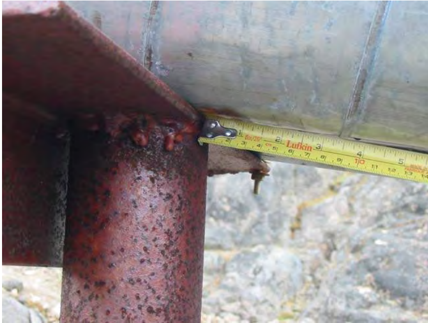
Photograph 7: Section of pipeline which is elevated above the ground and the pipe profile is steeper. The displacement in the photograph is approximately one inch.
