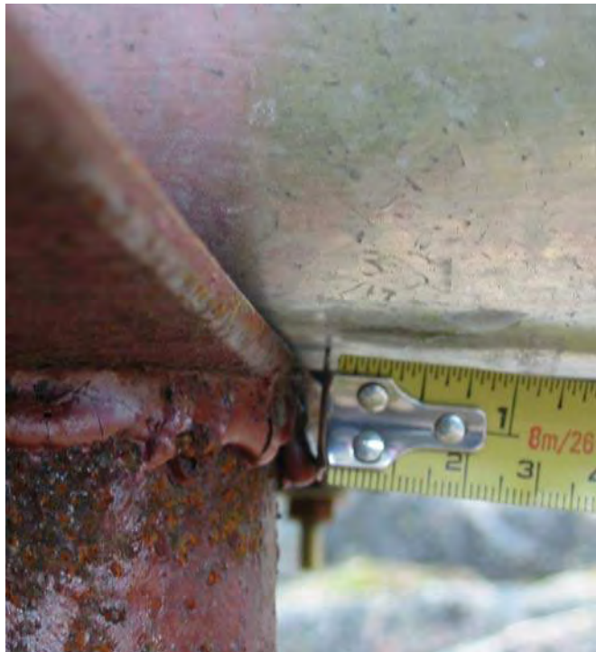
Photograph 6: Below the Heater House. The photograph illustrates a displacement of one inch. .
