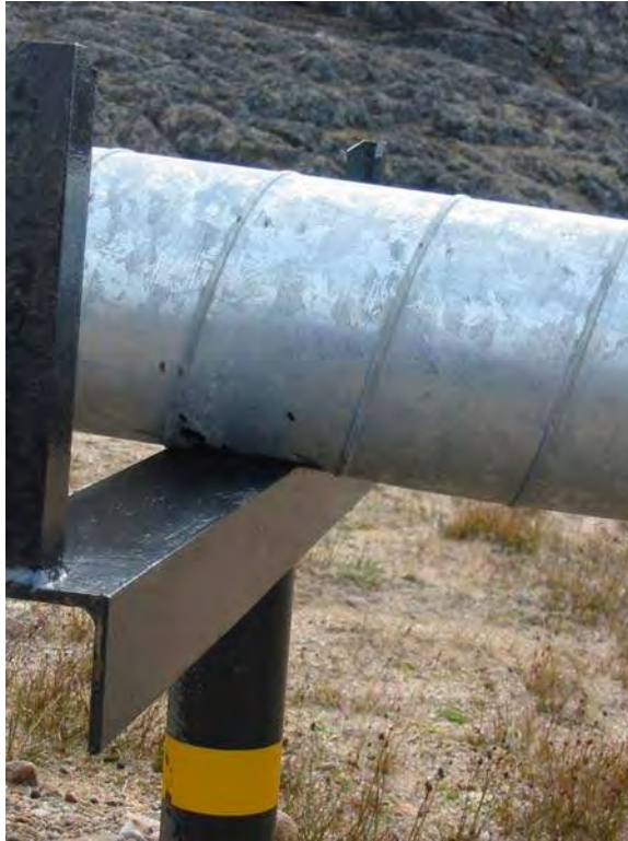
Photograph 13: Approximately 35 metres uphill from the expansion loop. Paint marks illustrate almost no movement of the pipeline at this location.
