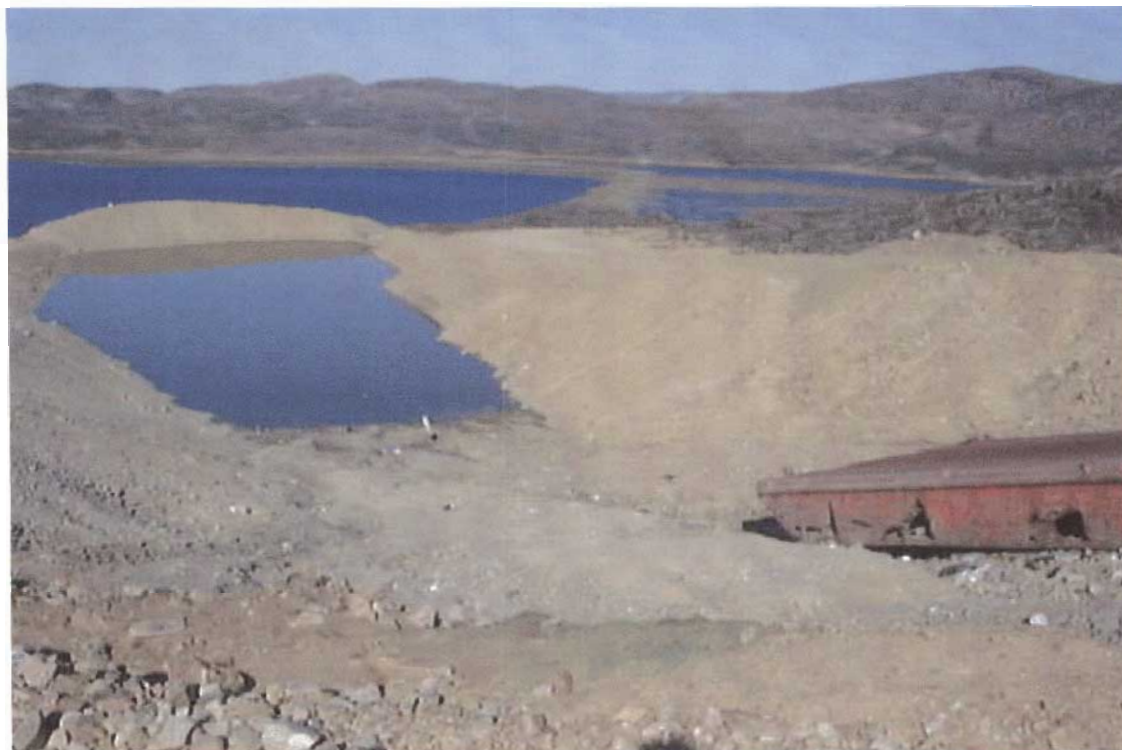
figure 1. Chute and first cell of the new sewage disposal facility; 2000/09/05.
