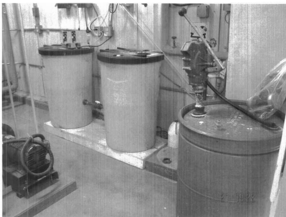
Figure 2. Chlorination system at the Cape Dorset pumphouse.
