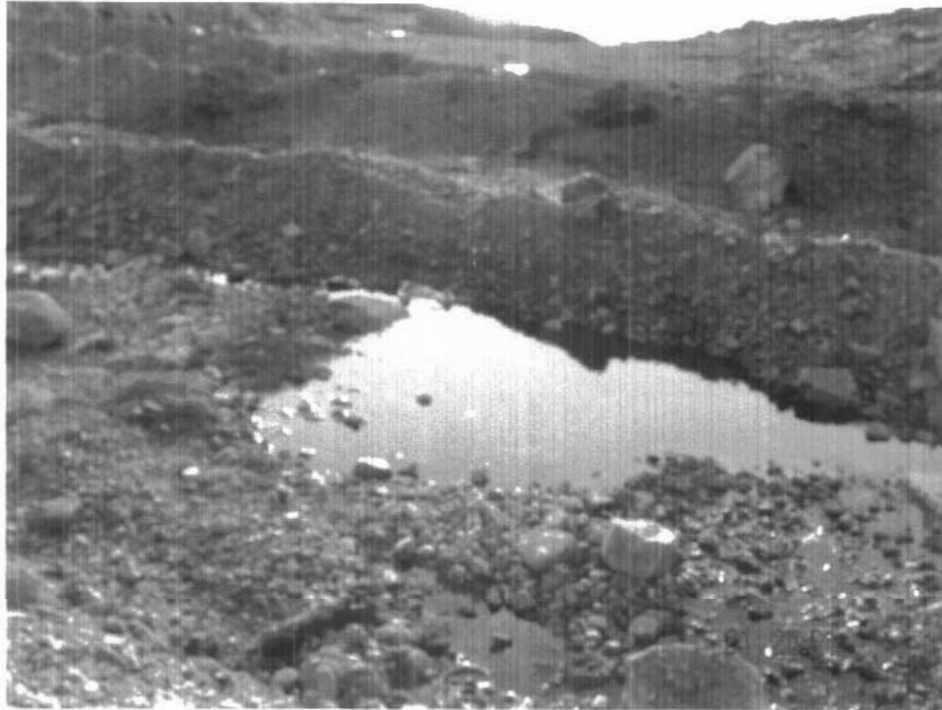
Figure 3. Berms placed between the old sewage lagoon in Cape Dorset and Telik Inlet to increase the lagoons "retention time".
