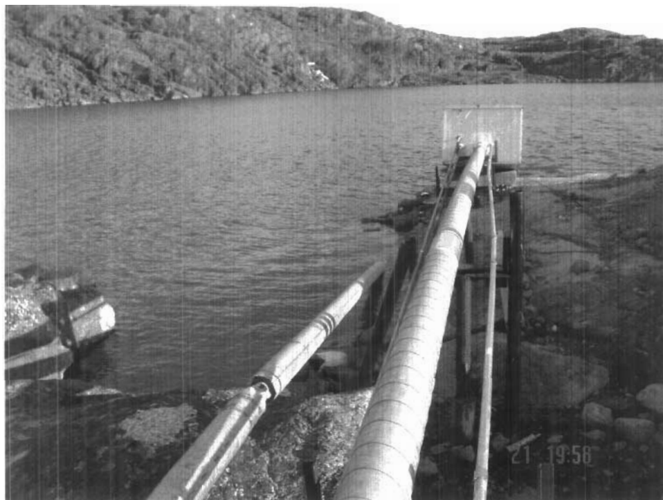
Figure 1. Cape Dorset pipeline running from Tee Lake to the municipal pumphouse.
