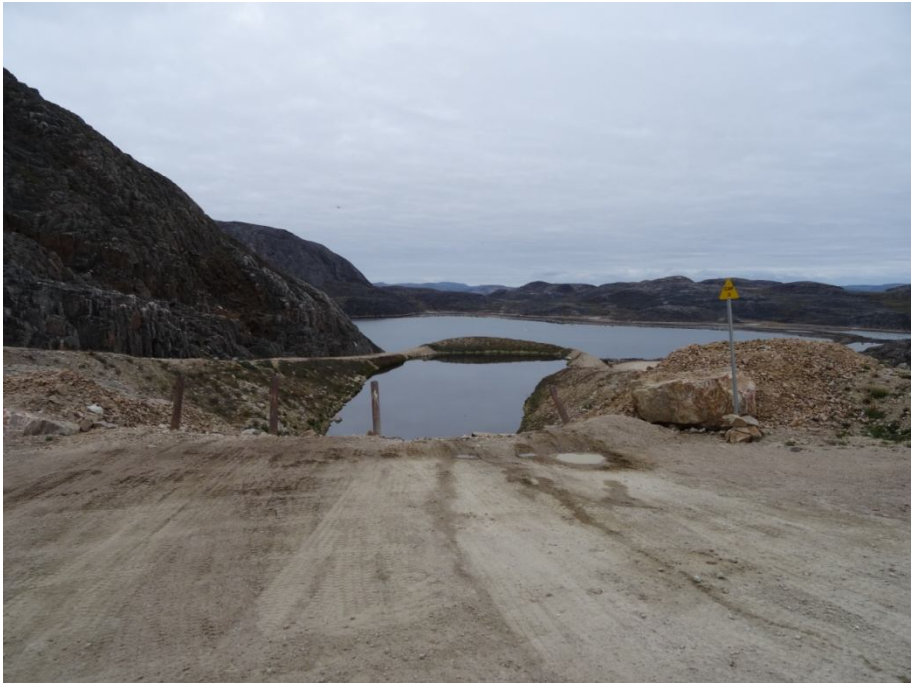
Figure 14 Lagoon Cell 1 of three tier lagoon system
