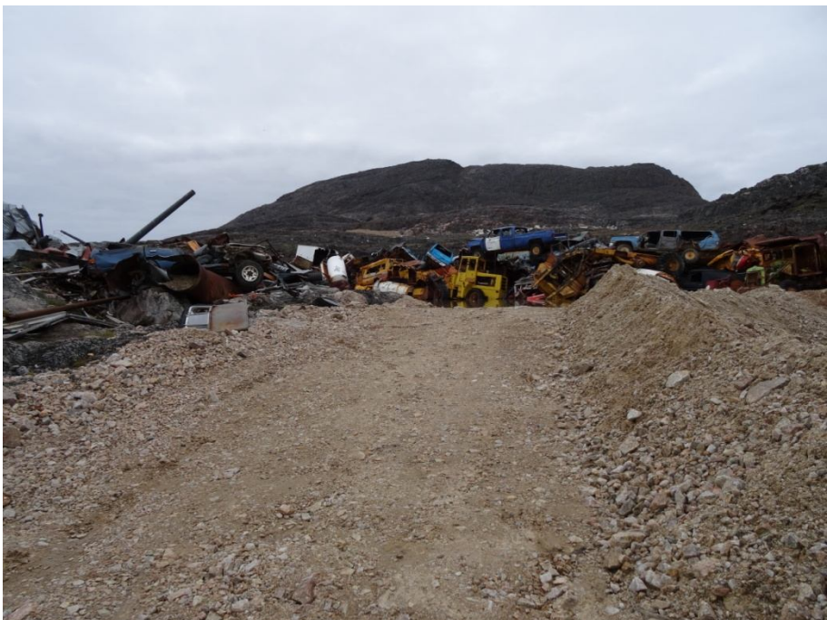
Figure 9 Berm slowing the flow of water off the Solid Waste Management Area
