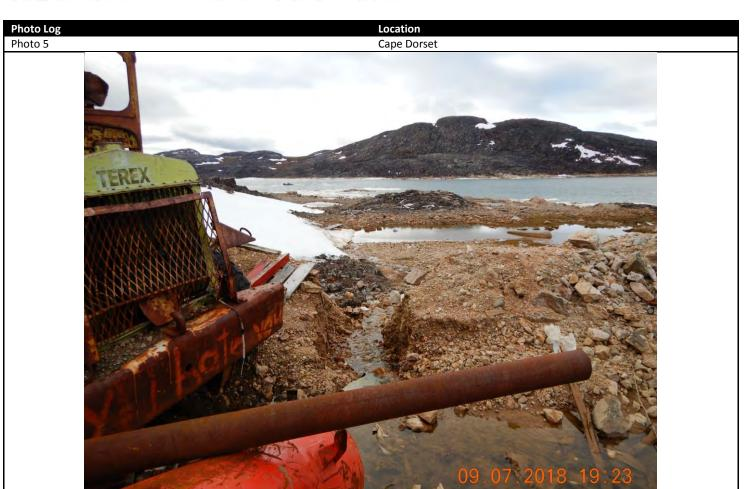
Description: erosion of the containment wall to mitigate any leachate from the bulk metal section has eroded, and compromised its intended purpose.
