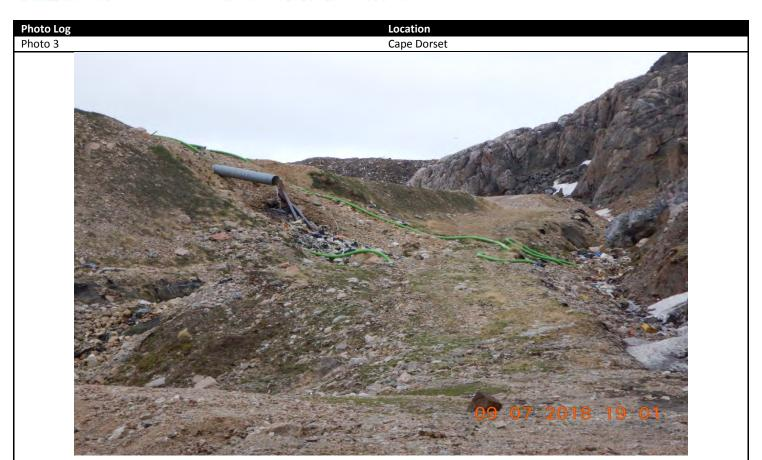
Description: signs of overflow and migration to drainage ditch south side of sewage lagoon cell.
