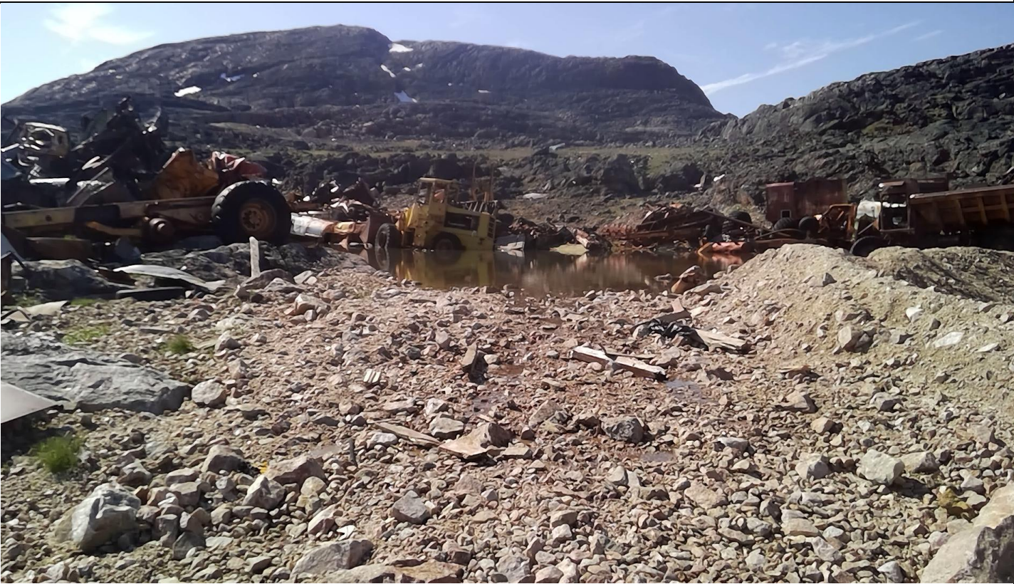
Description: A berm rebuilt into the solid waste facility is overflowing. The water being built up has to be tested and treated if found to have contaminants before being released.
