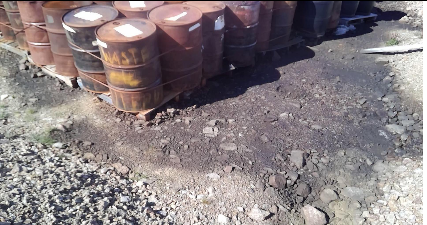
Description: Observable spill within the 3 walled berm for hazardous waste drums.
