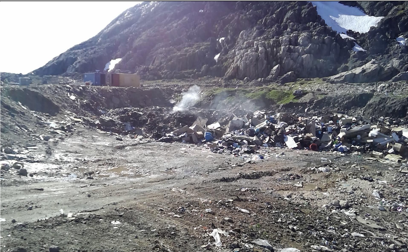
Description: Fencing at the burn and cap section of the solid waste facility. Fencing condition has been demolished.
