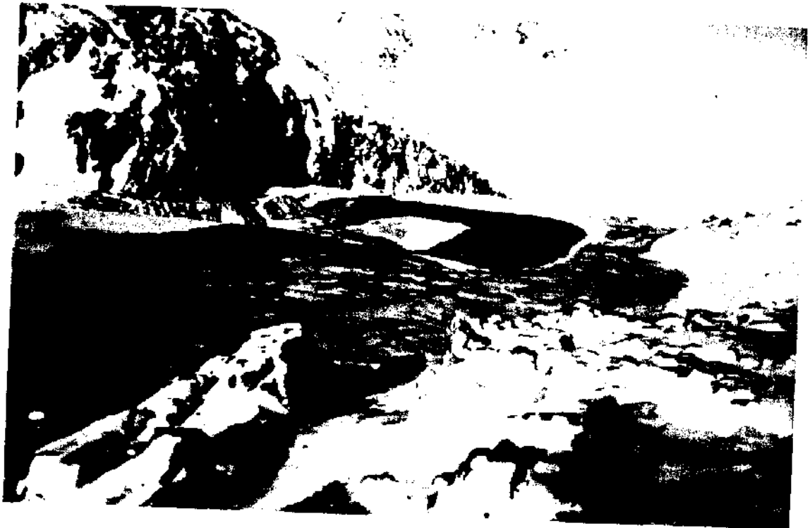
View of Cells #2 and #3 with Sewage Running Over Ice Cover (April 2003)
