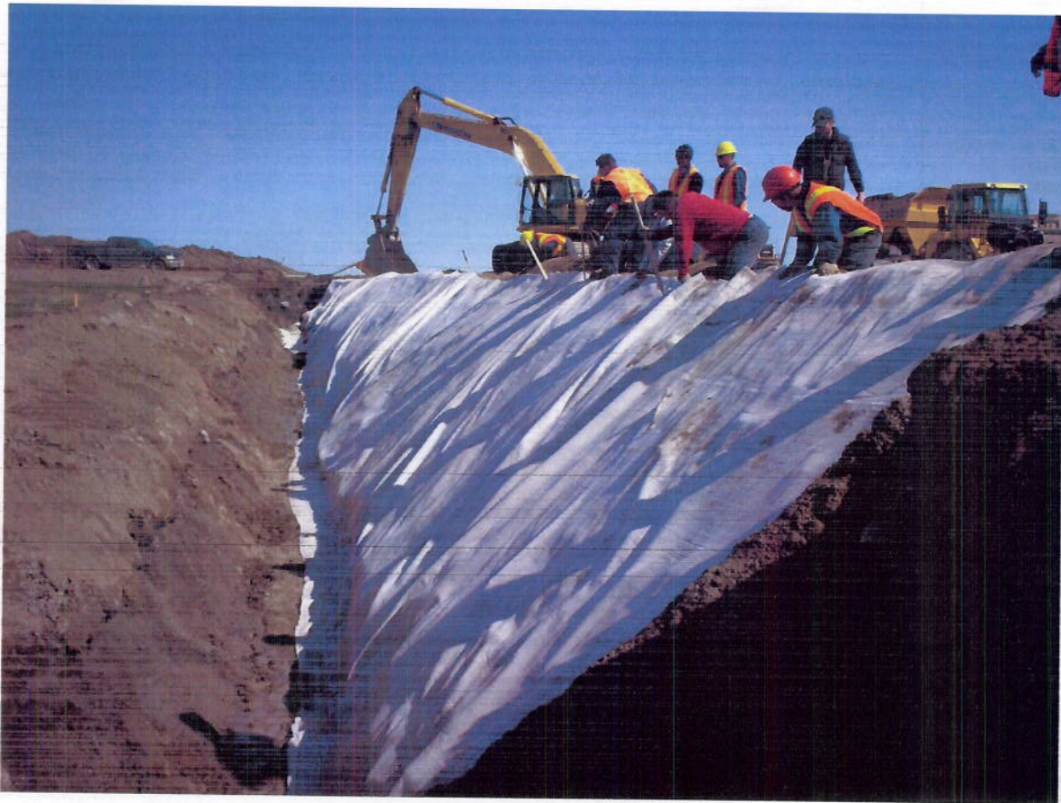
Image 5.3.1 Liner Installation
