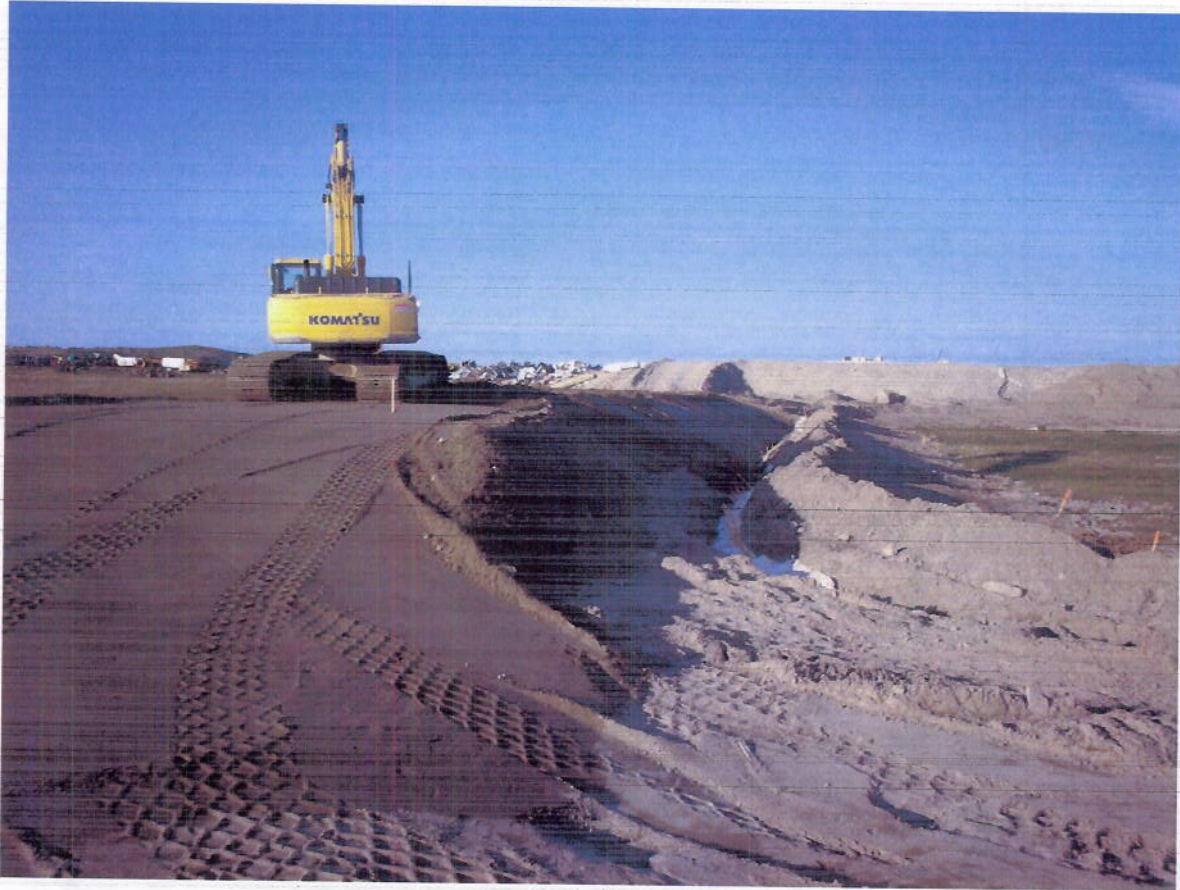
Image 5.2.1 Berm Construction
