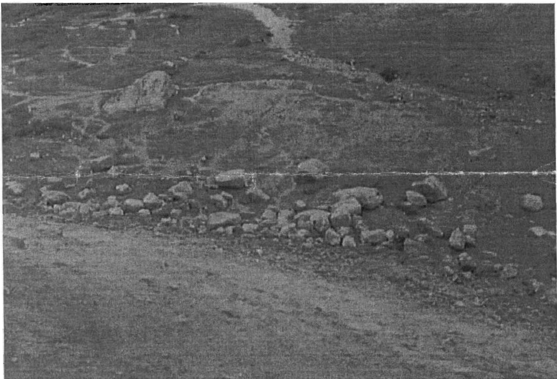
figure 3. Veins of seepage along the toe of the sewage lagoon; 2000/08/17.
