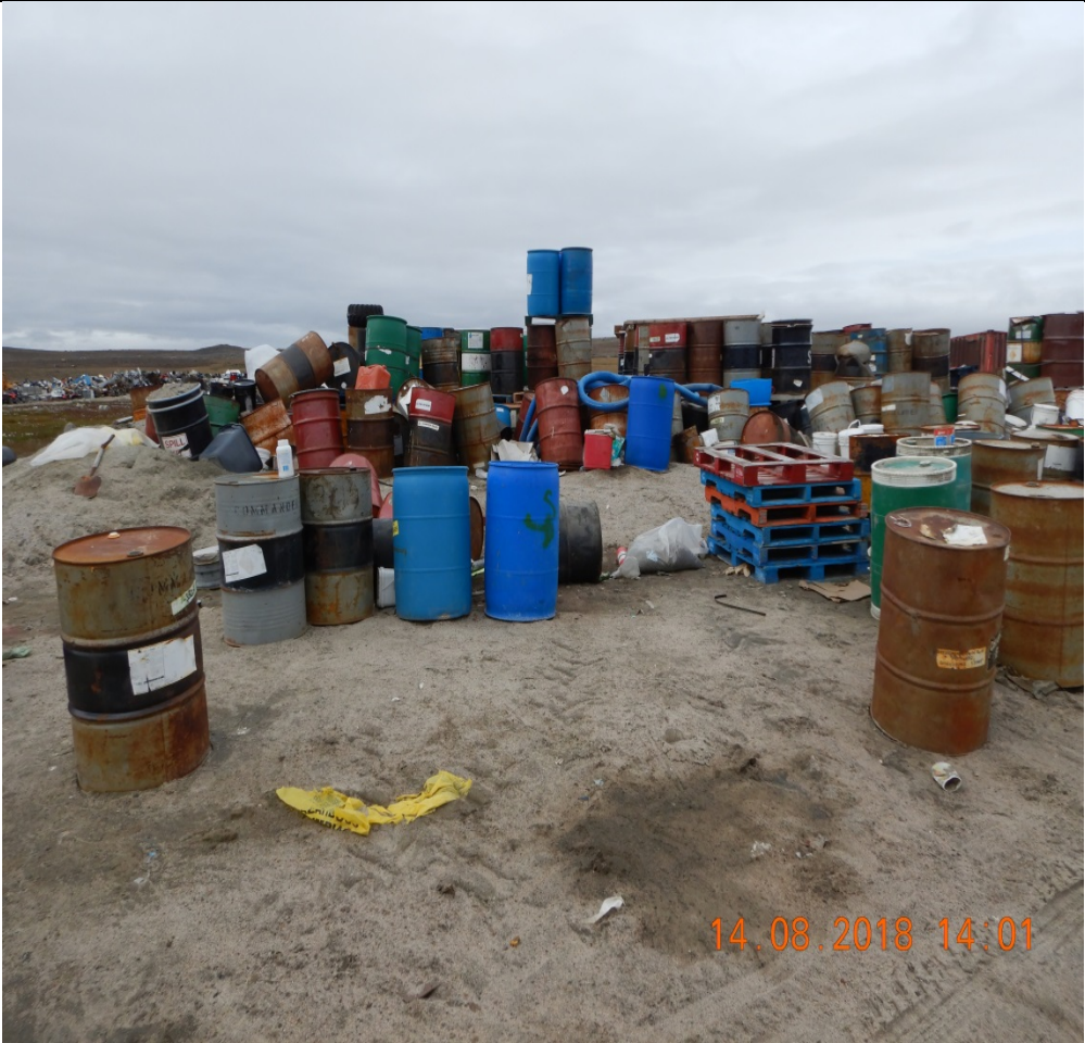
Description: Hazardous Waste Berm – overfilled with waste oil drums. Waste oil drums deposited outside of bermed area. Signs of spills on ground outside of the bermed area.
