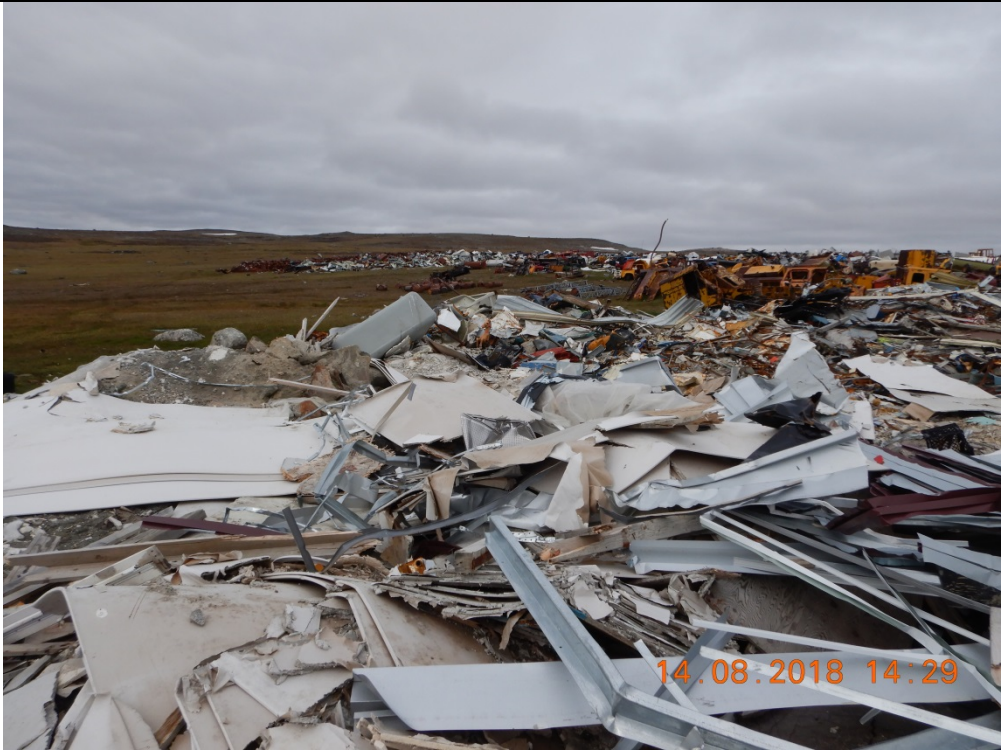
Description: the outer extent of bulk metal section of land farm, no berm to mitigate any potential deposit of wastes onto environment
