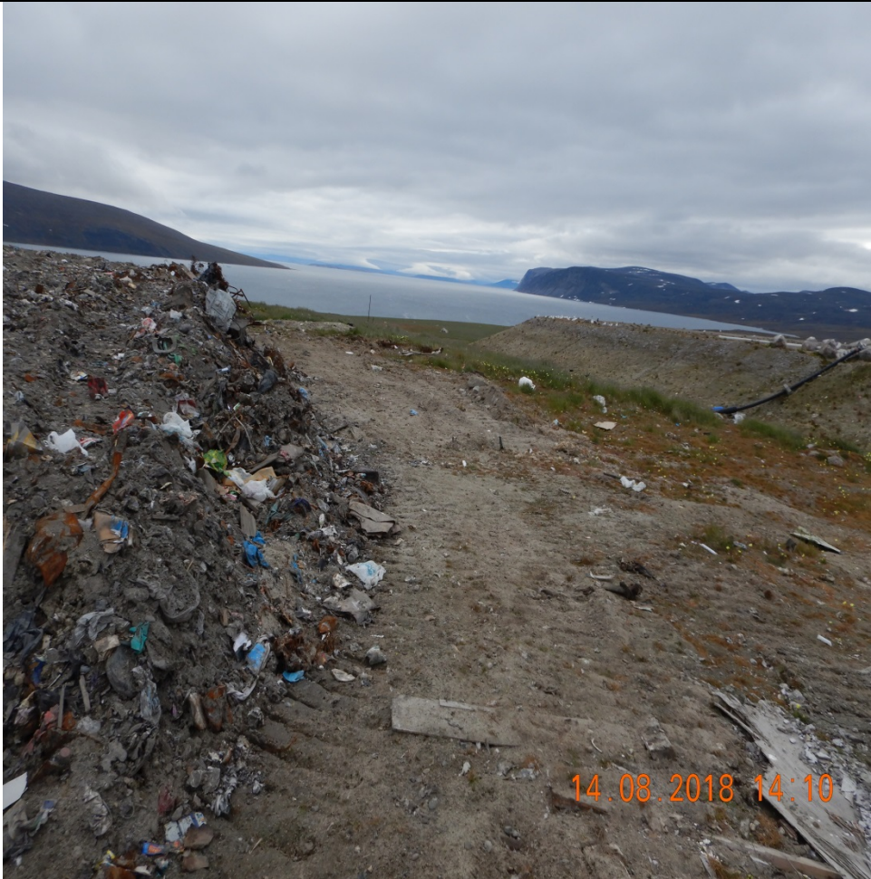
Description: Fire Pit – No fencing on East Side, wind may blow ash and debris out of area onto the environment, the ocean, and to the sewage lagoon
