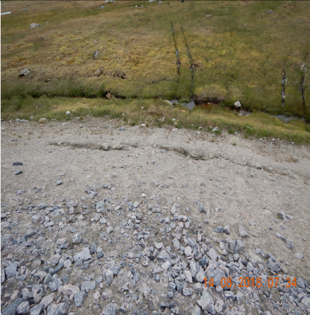
Description: base of sewage lagoon walls appears to be slumping
