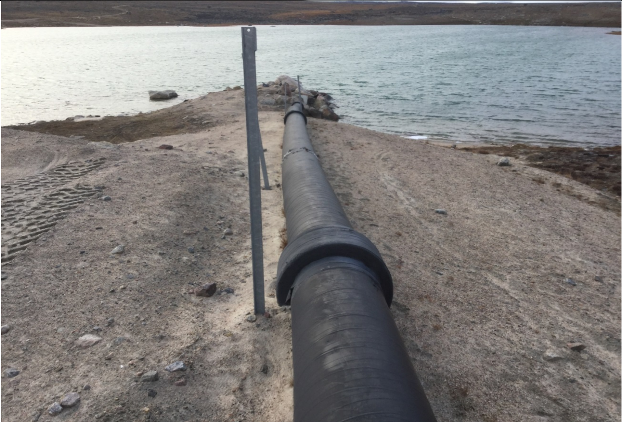
Description: Water Source Lake. Water Extraction pipe
