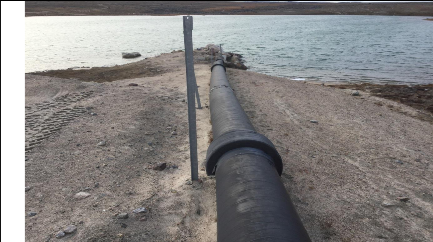
Description: Water Source Lake. Water Extraction pipe. Similar in design as the Pond Inlet Water Pump House
