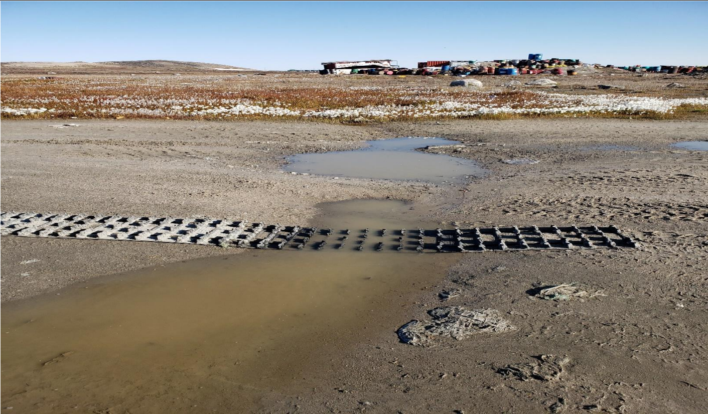
Description: What was observed as a puddle along the side of the road between the Bulk Metal and the Hazardous Waste Facility has turned into a seasonal surface water creek that takes water from the Hazardous Waste Facility to through the Bulk Metal section of the Solid Waste Facility.
