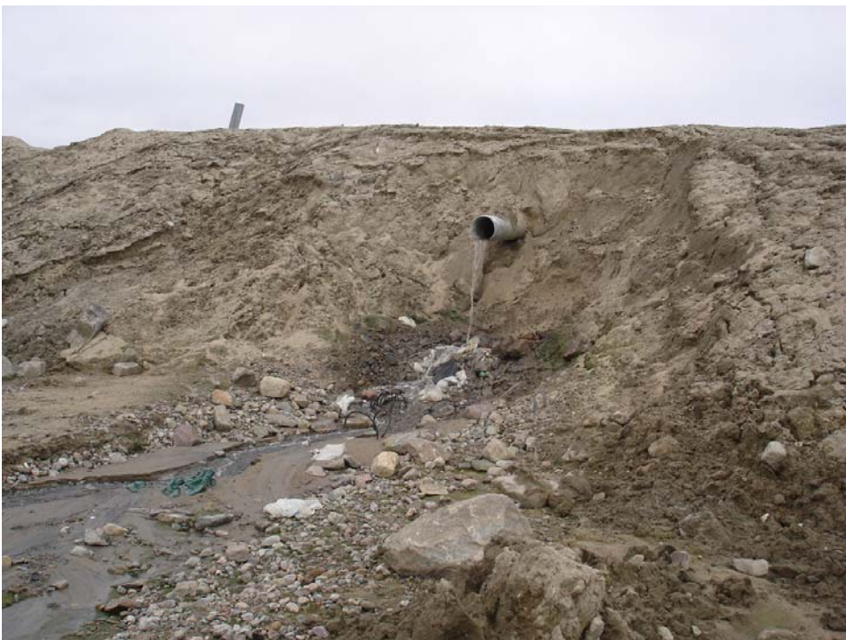
Figure A-8: West berm of existing lagoon with overflow pipe, showing berm erosion
