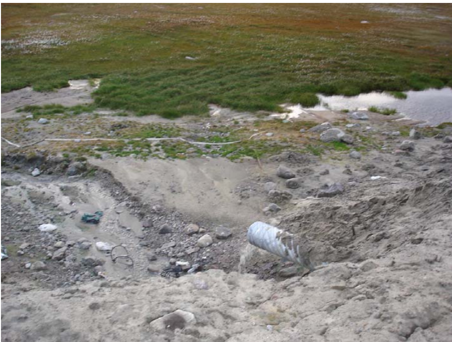
Figure A-6: Overflow pipe in west berm of existing lagoon
