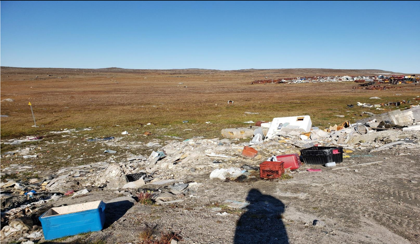
Description: the outer extent of bulk metal section of land farm, no berm to mitigate any interaction with external environmental elements, and migration of wastes outside the facilities. A monitoring station is observed in left hand side midground.
