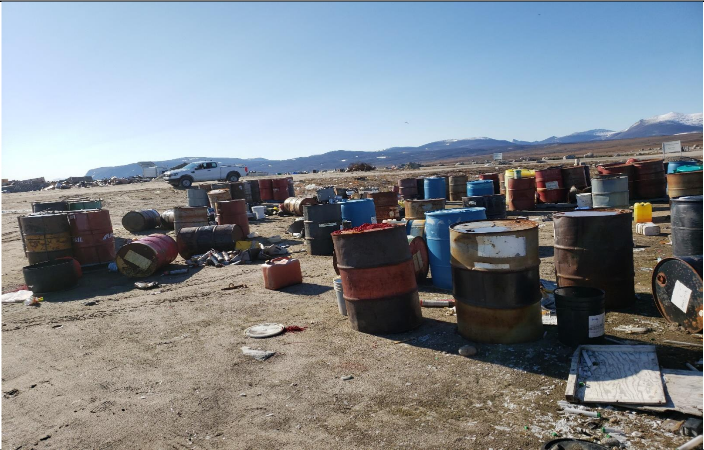
Description: Hazardous Waste Disposal Facility. Berm is overfilled with waste oil drums. Waste oil drums deposited outside of bermed area.
