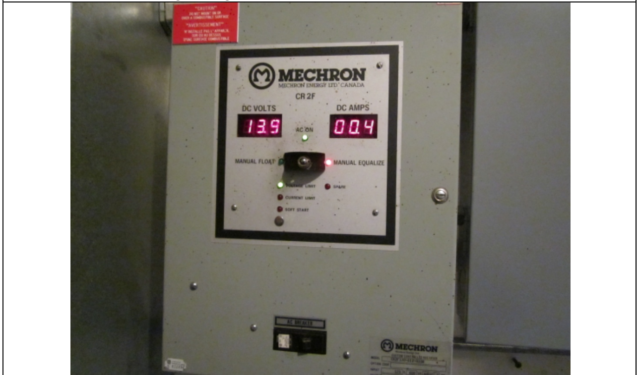
Photo 10 – Generator Battery Charger
