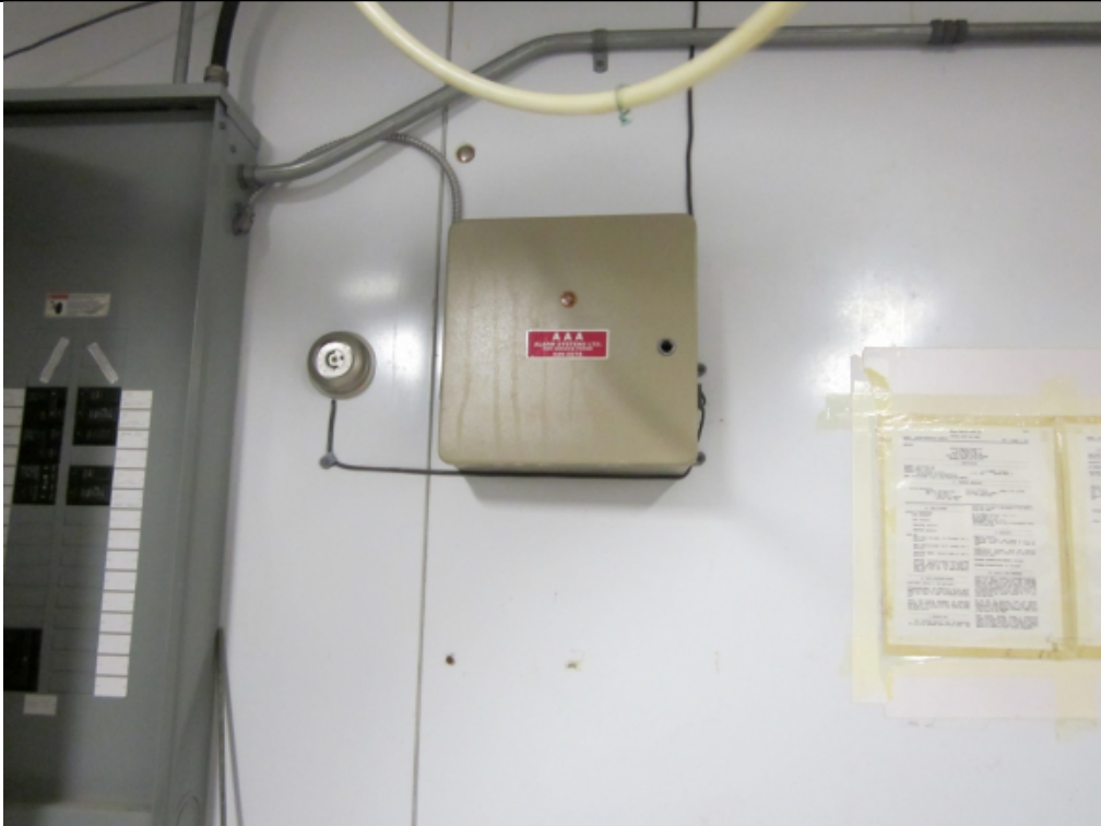
Photo 41 – Truck Fill Station Alarm Panel
