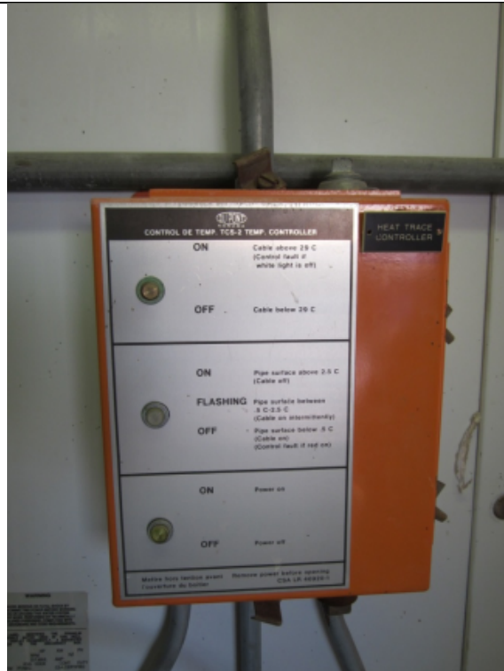
Photo 31 – Heat Trace Controller Enclosure
