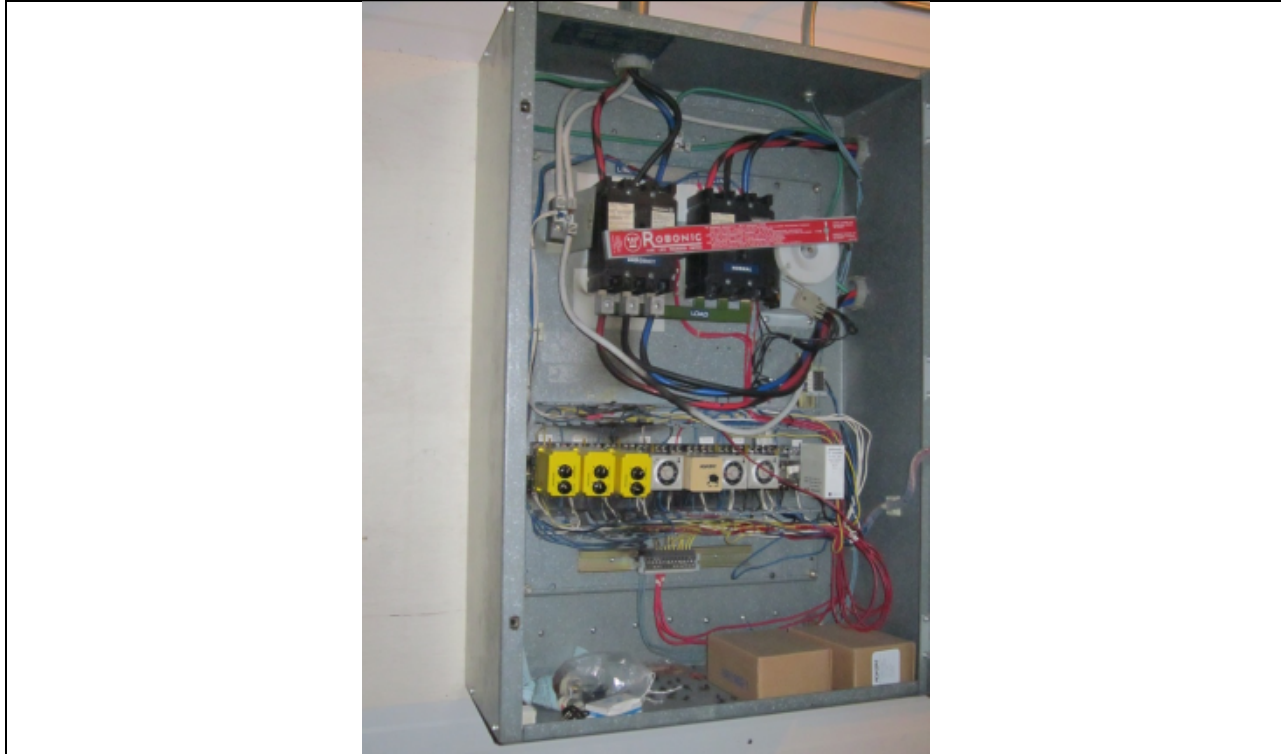
Photo 7 – Interior of Automatic Transfer Switch with Visible Damage
