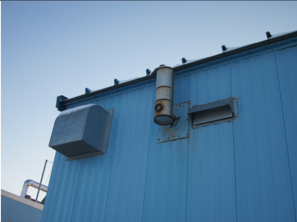
Photo 13 – Generator Exhaust Pipe Exterior
