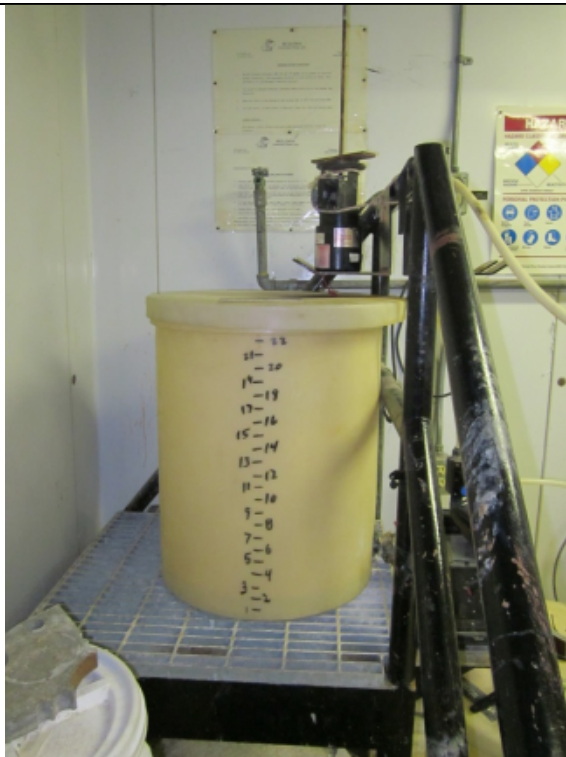
Photo 34 – Truck Fill Station Chlorine Mixer
