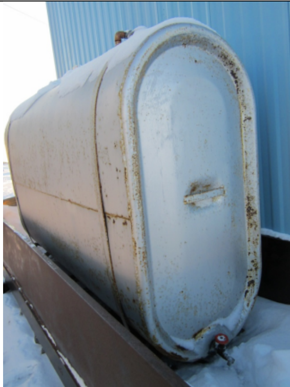
Photo 14 – Generator Outdoor Fuel Tank
