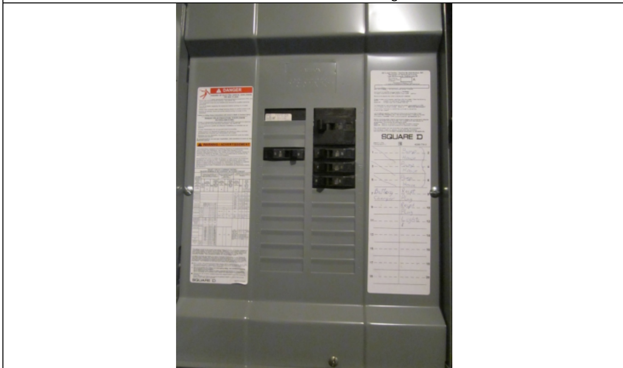
Photo 8 – Generator Building Subfeed Panel to Truck Fill Station
