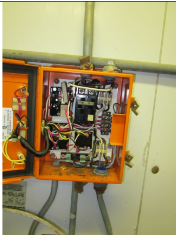
Photo 32 – Interior of Pump P1 Heat Trace Controller
