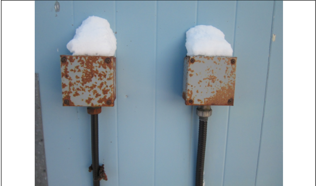
Photo 21 – Exterior Junction Boxes for Electrical Service to Truck Fill Station
