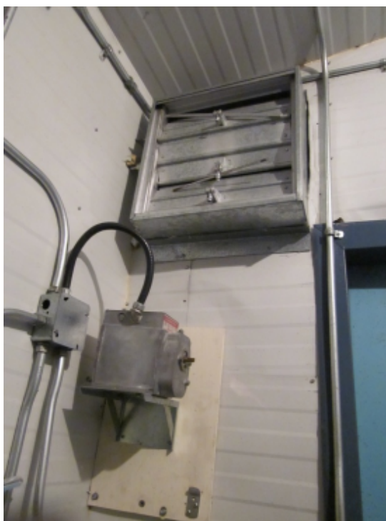
Photo 12: Unserviceable Intake Damper
