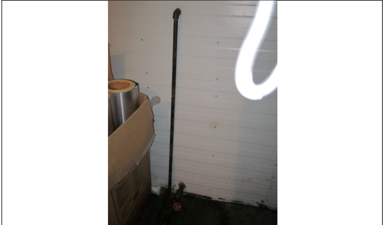
Photo 17 – Fuel Line to Generator
