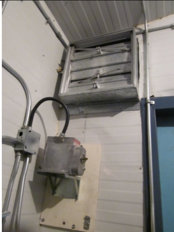
Photo 11 – Generator Air Intake Damper
