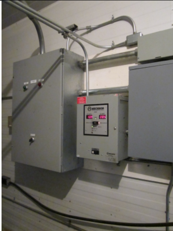
Photo 5 – Automatic Transfer Switch and Battery Charger
