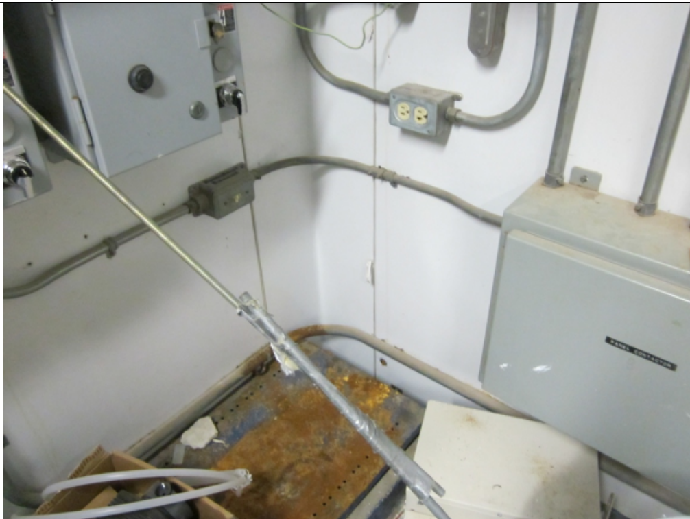
Photo 28 – Corroded Power Supply Conduit in Corner of Station
