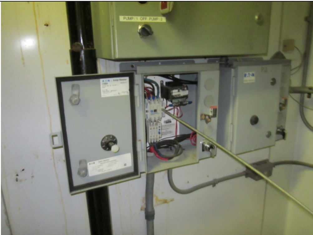
Photo 26 – Pump P1 Starter in Operation with Steel Rod Blocking Trip Unit
