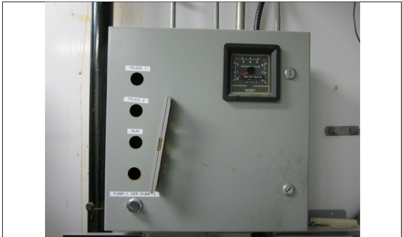
Photo 35 – Pump Controller and Relay Panel with Missing Push Buttons
