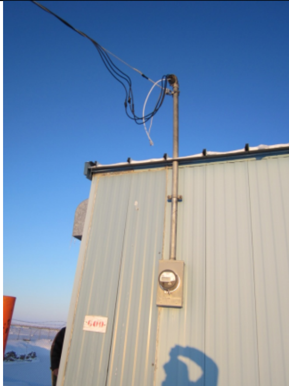
Photo 3 – Generator Building Electrical Supply
