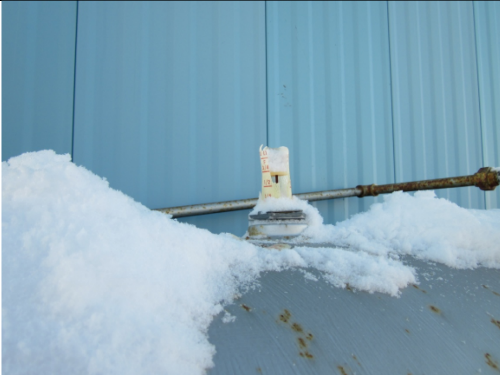
Photo 15 – Broken Fuel Tank Level Meter
