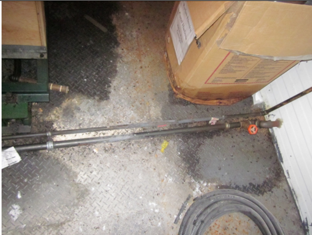
Photo 18 – Fuel Line to Generator with Signs of Leaking
