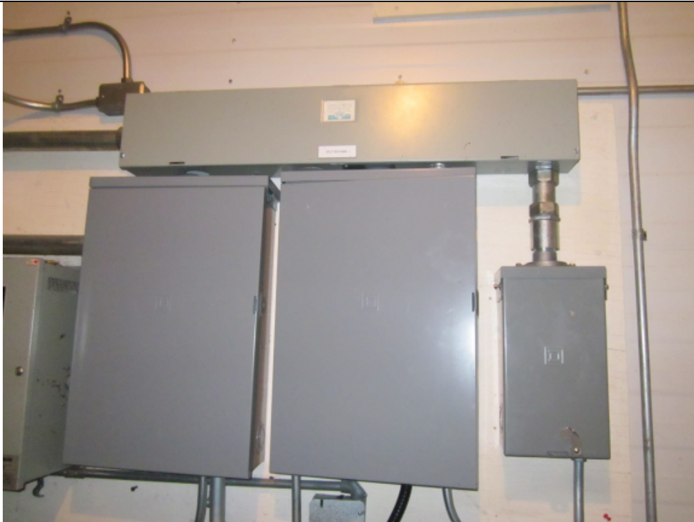
Photo 4 – Main Disconnect, Splitter and Panels
