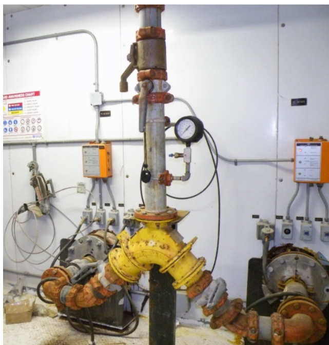
Photo 6: Supply Piping Entry
