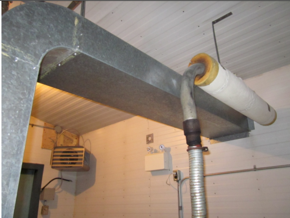
Photo 12 – Generator Ducted Exhaust Interior
