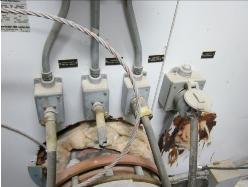
Photo 29 – Pump P1 Receptacle and Separating Flexible Plug with Exposed Wiring on Right. Heat Trace Connections to Pump P1 with Removed/Broken Control Connection
