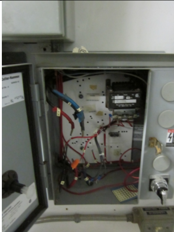
Photo 27 – Pump P2 Starter Enclosure without Starter
