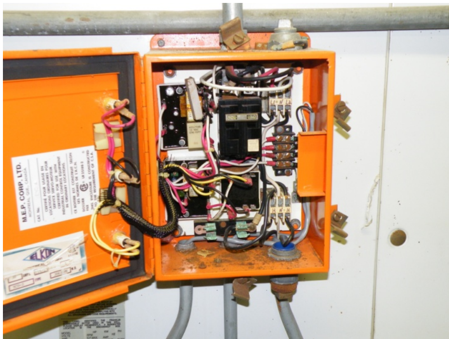
Photo 9: Heat Trace Controller Internal Conditions
