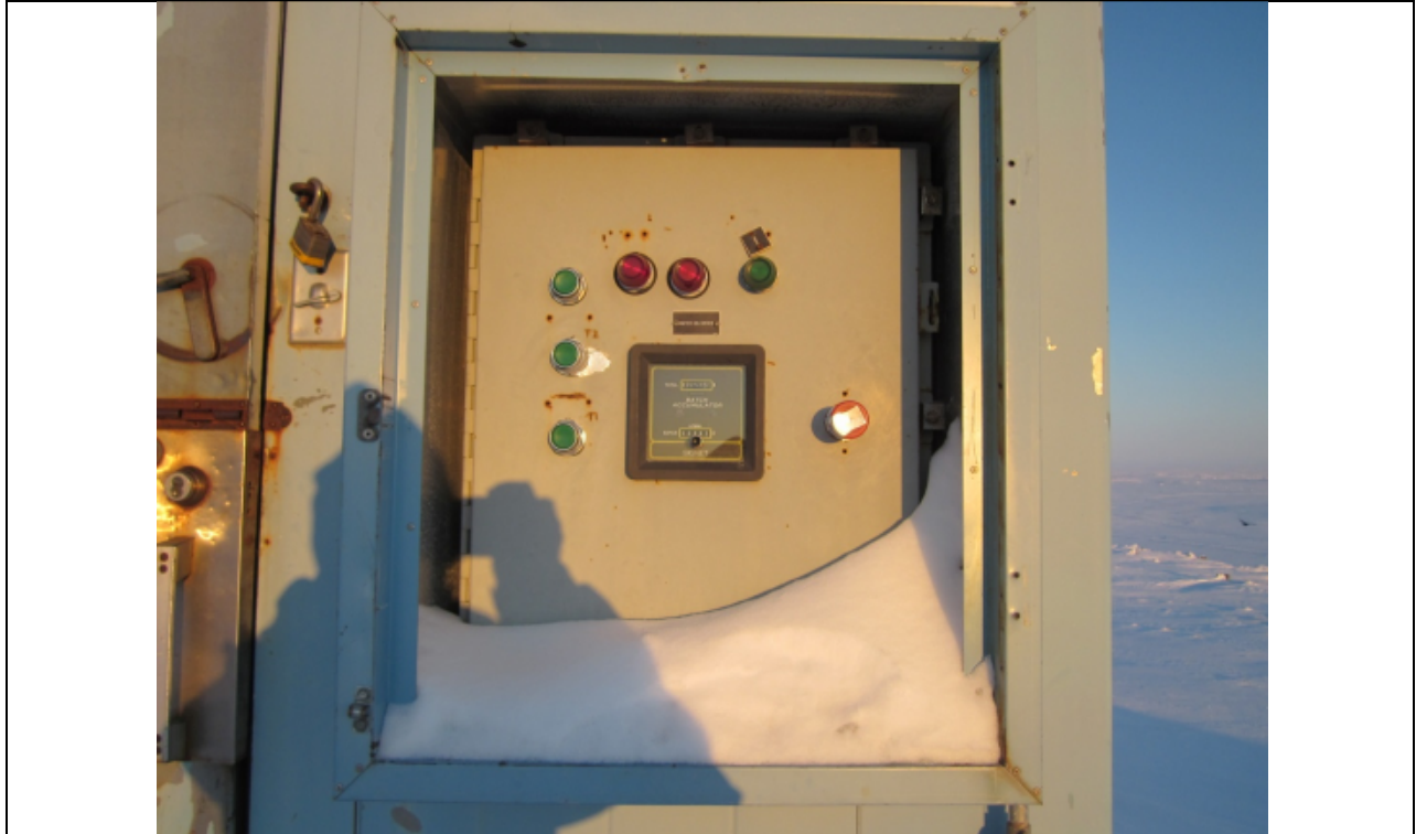
Photo 37 – Exterior Pump Controls
