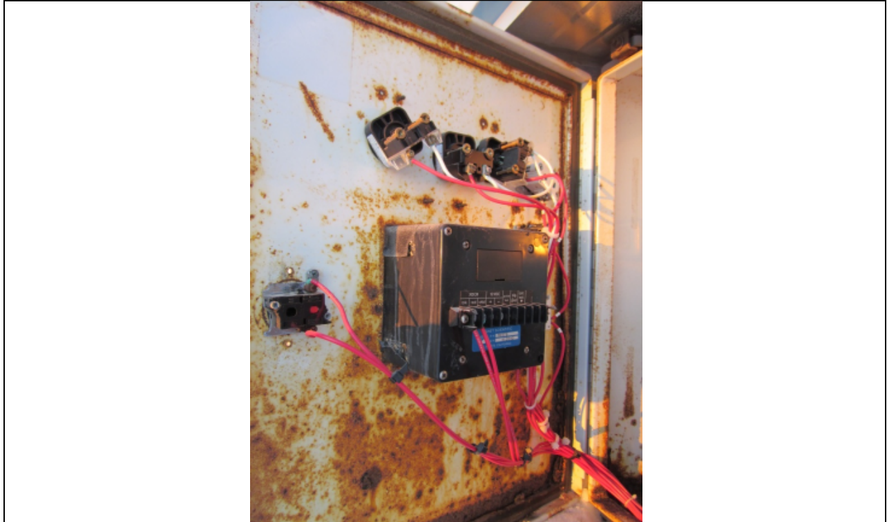
Photo 39 – Exterior Pump Controller Door Mounted Devices
