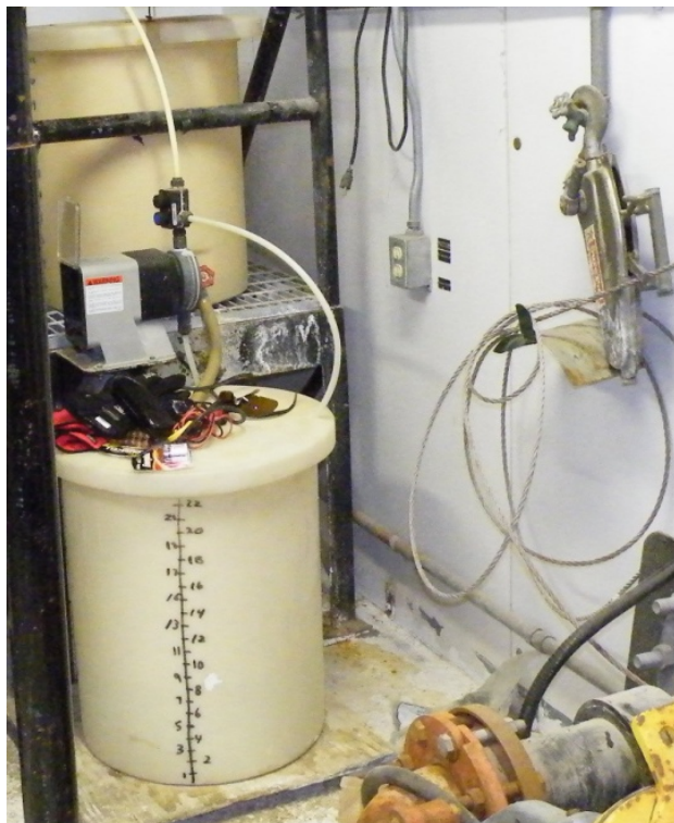
Photo 5: Chlorine Tank and Metering Pump
