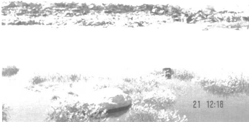
Figure 5. Ponding at the toe of the Coral Harbour landfill.
