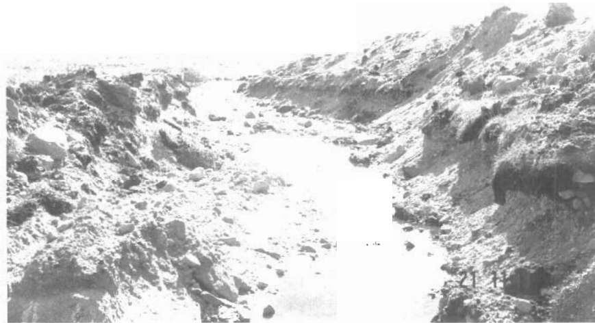
Figure 9. Drainage ditch for Coral Harbour sewage effluent flowing from the lagoon and overland to the first pond.
