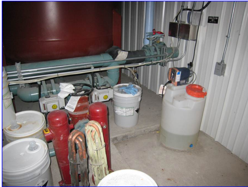
Photograph No. 19 Chlorination station.
