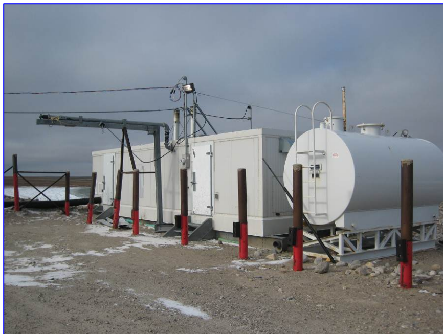
Photograph No. 16 View of water pumping station, emergency truck fill station, and fuel tank.
