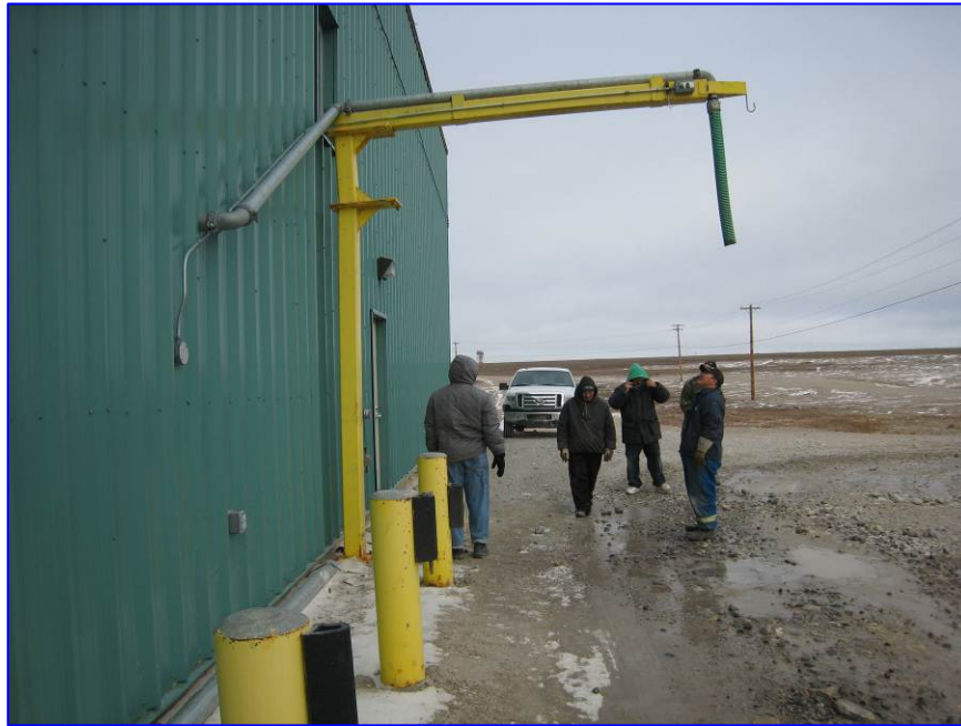
Photograph No. 21 Truck fill station.
