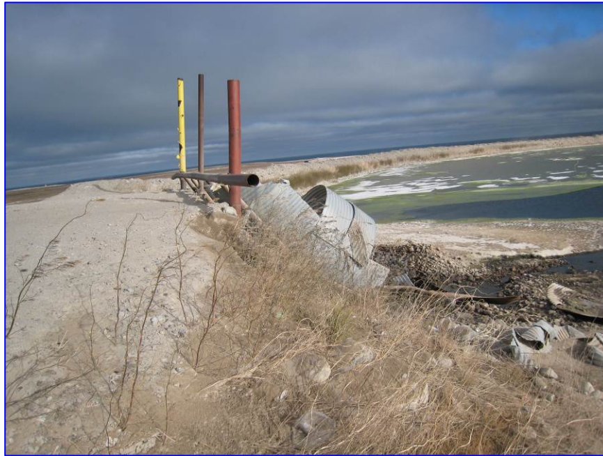
Photograph No. 7 Discharge chute. Note erosion at toe of berm.
