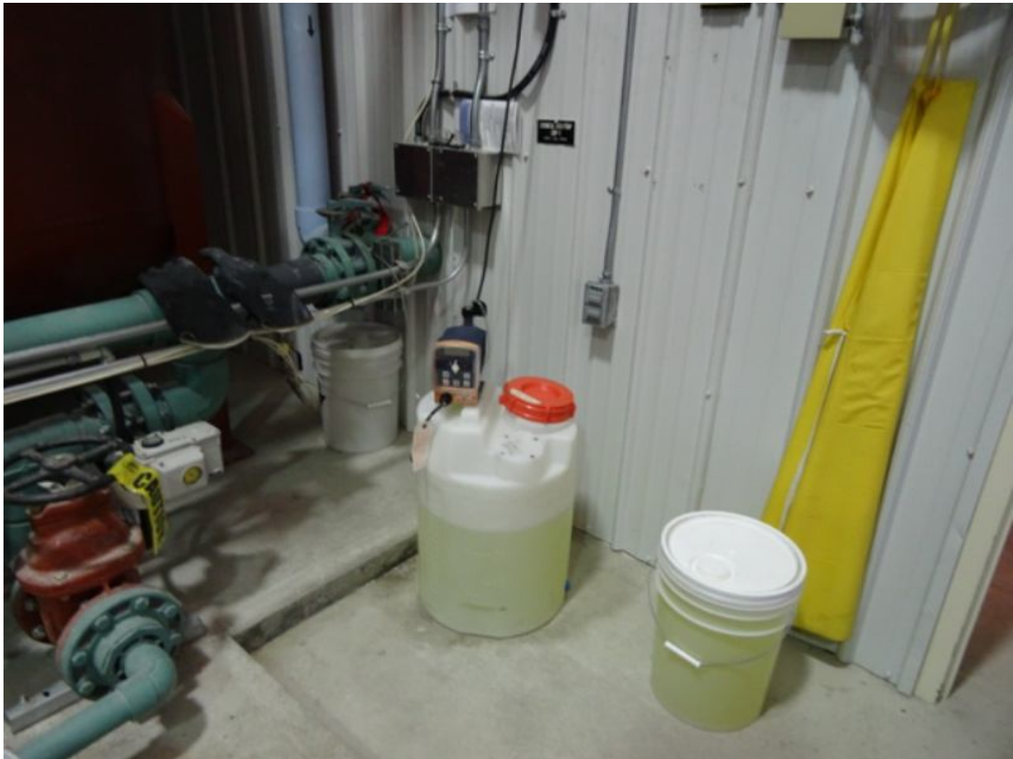
Figure 7 Chlorine station # 2 at Truck fill station
