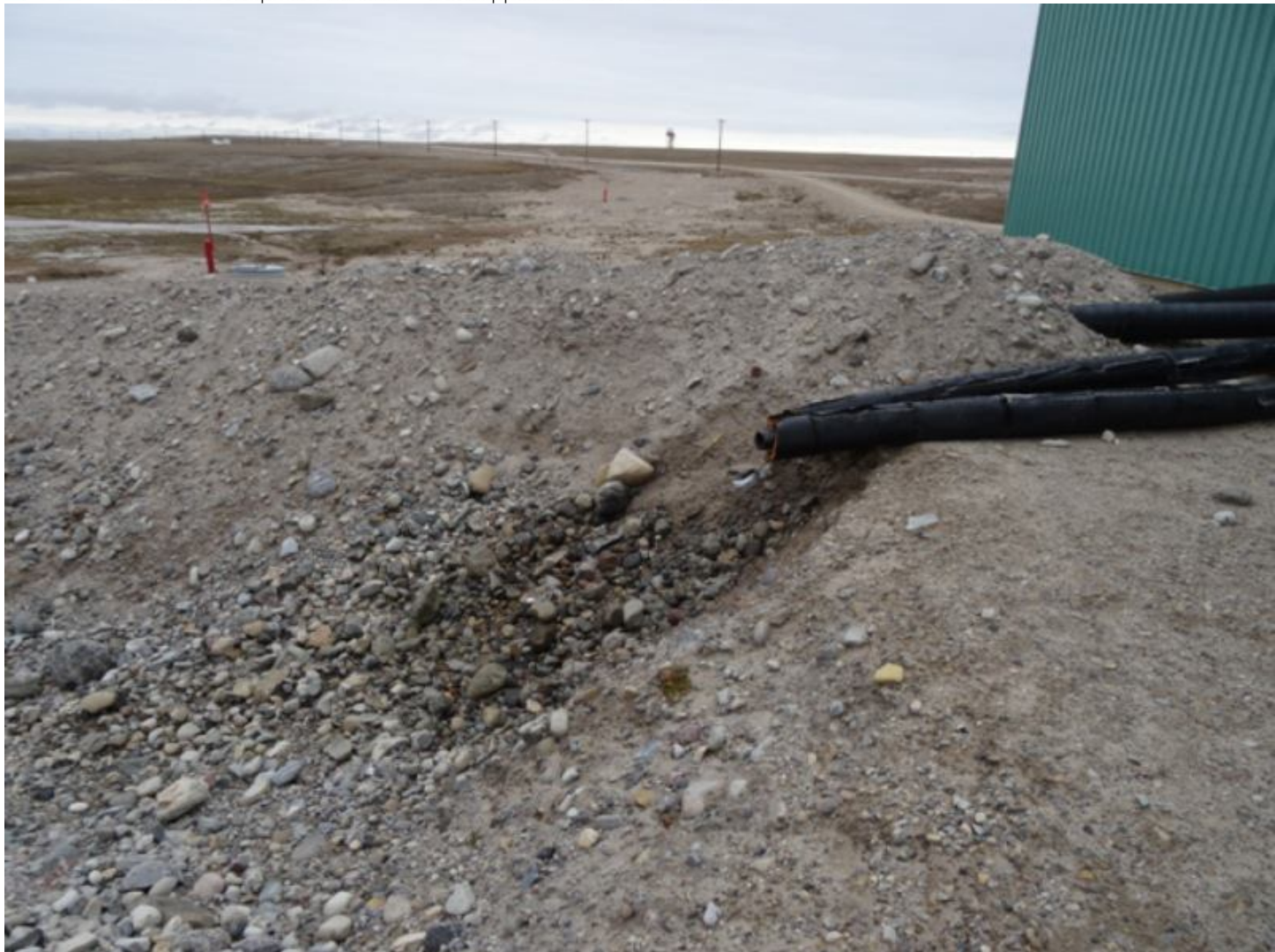
Figure 4 Piped in Diversion for Direct Discharge from Truck fill building
