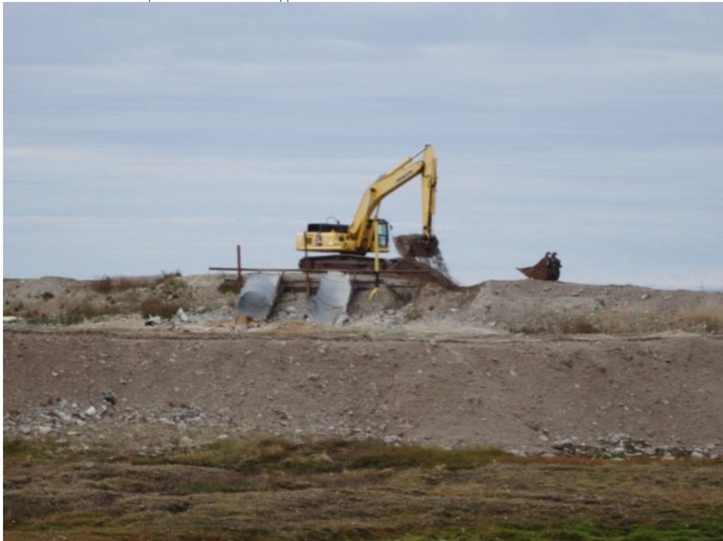
Figure 10 Excavator at truck drop off taking out berm wall material
