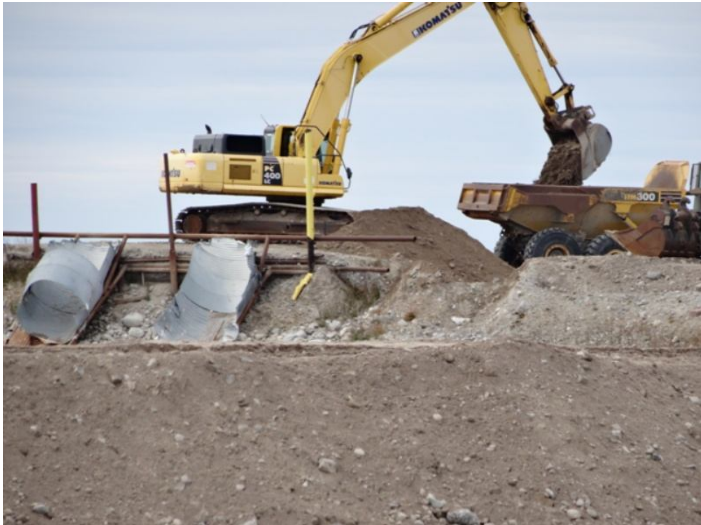
Figure 11 Excavator taking down berm wall at truck drop off
