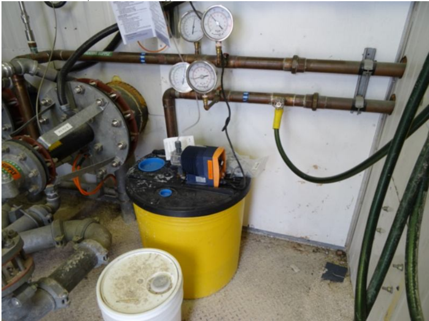
Figure 2 Chlorine tank and pump in in-take/ pumping station
