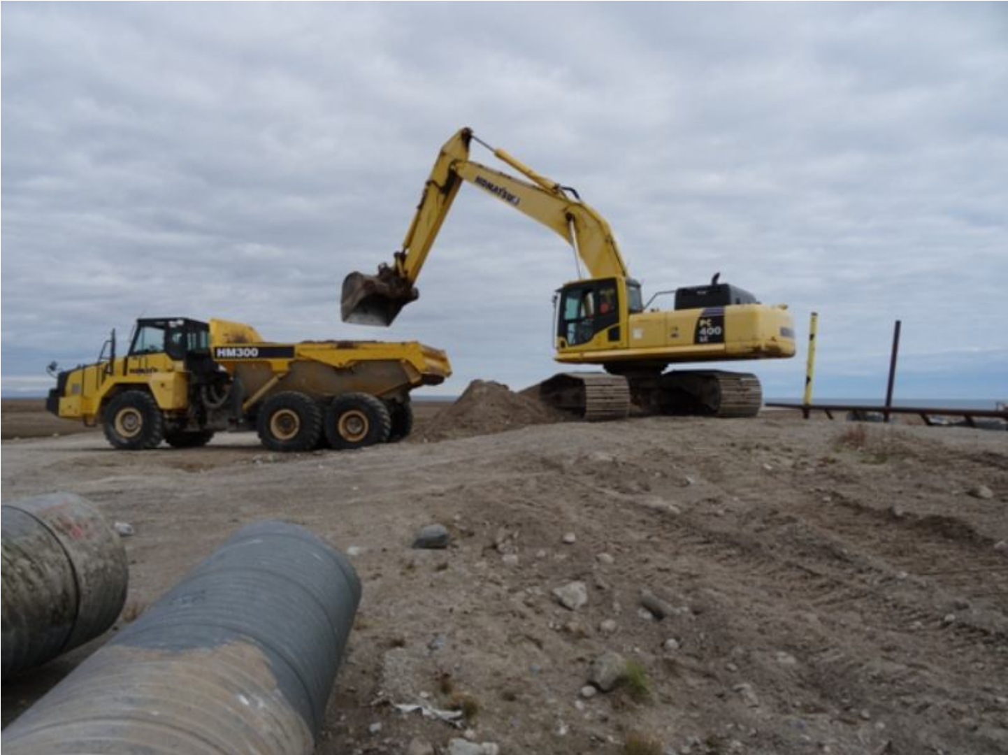
Figure 9 Excavator taking down lagoon wall
