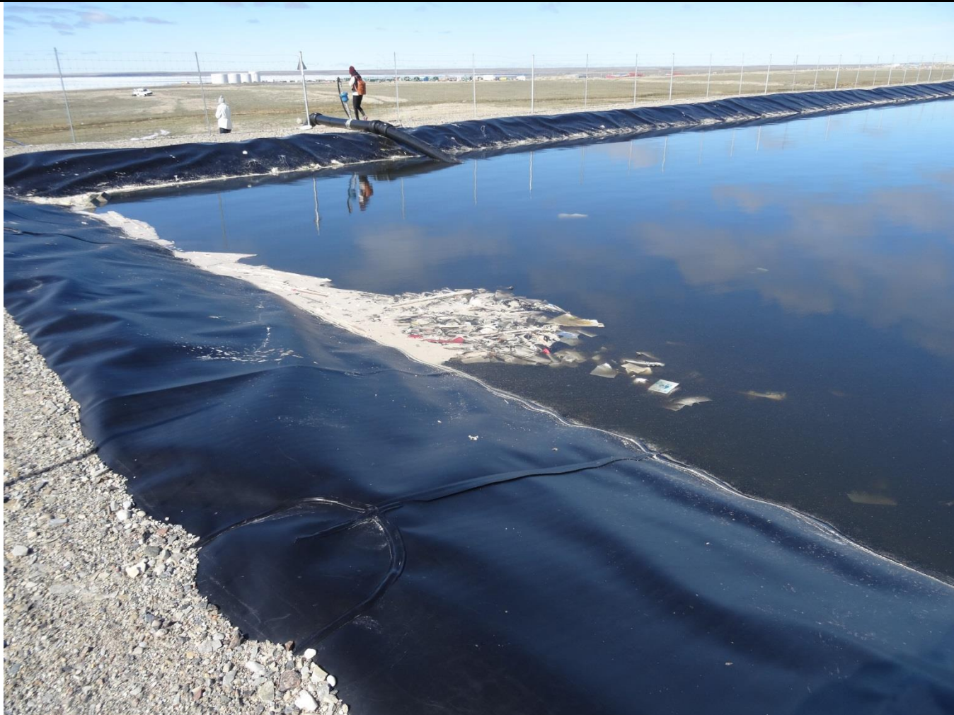
Description: Sewage Lagoon showing high level of Liquid Contents and Floating Debris – July 13 th
