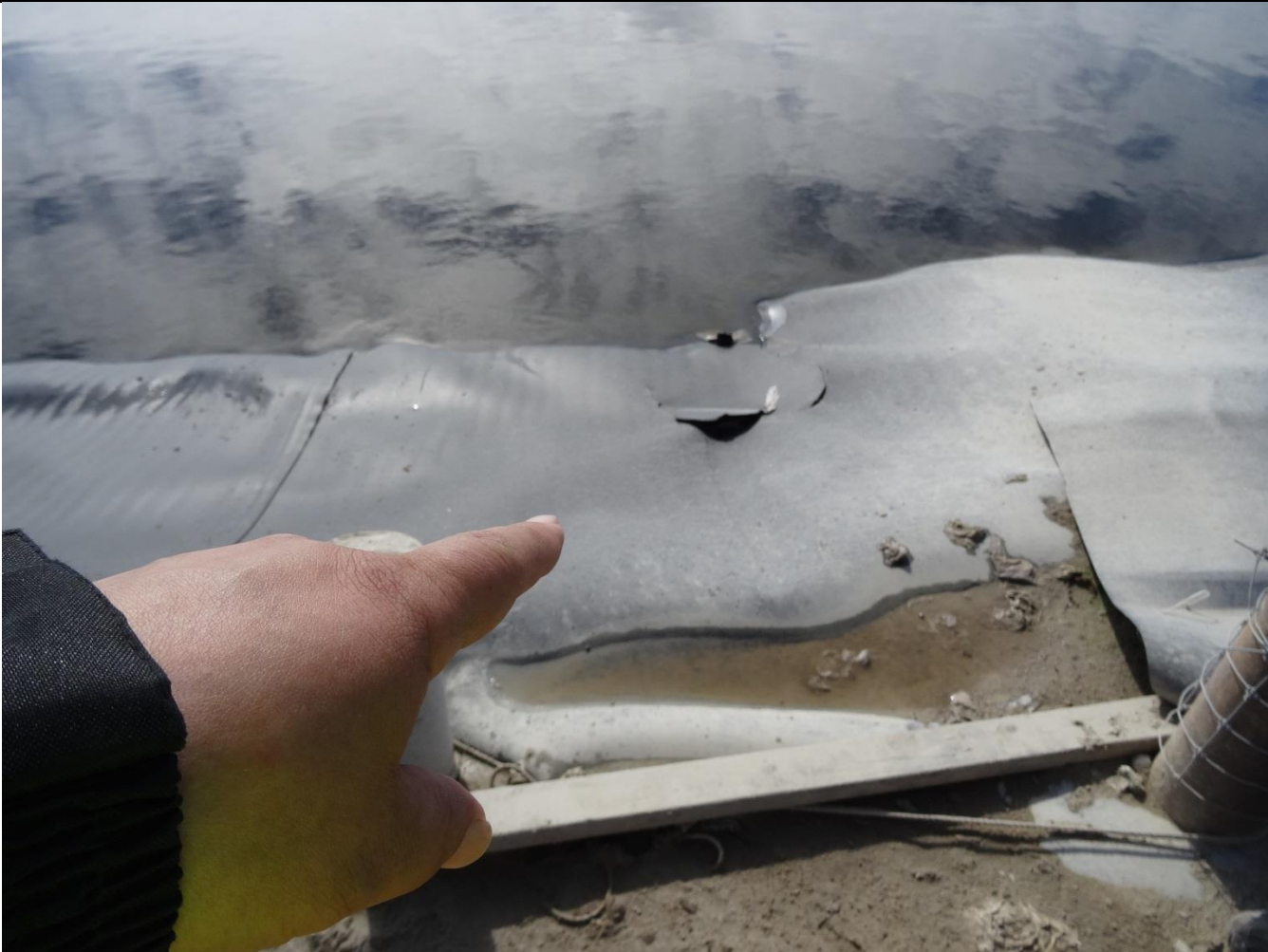
Description: Tear #3 and #4 in Sewage Lagoon Liner at Truck Dumping Location requiring Repair after Decanting – July 13 th
