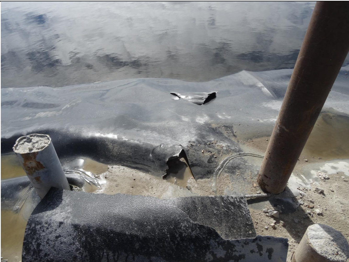
Description: Tear #1 and #2 in Sewage Lagoon Liner at Truck Dumping Location requiring Repair after Decanting – July 13 th
