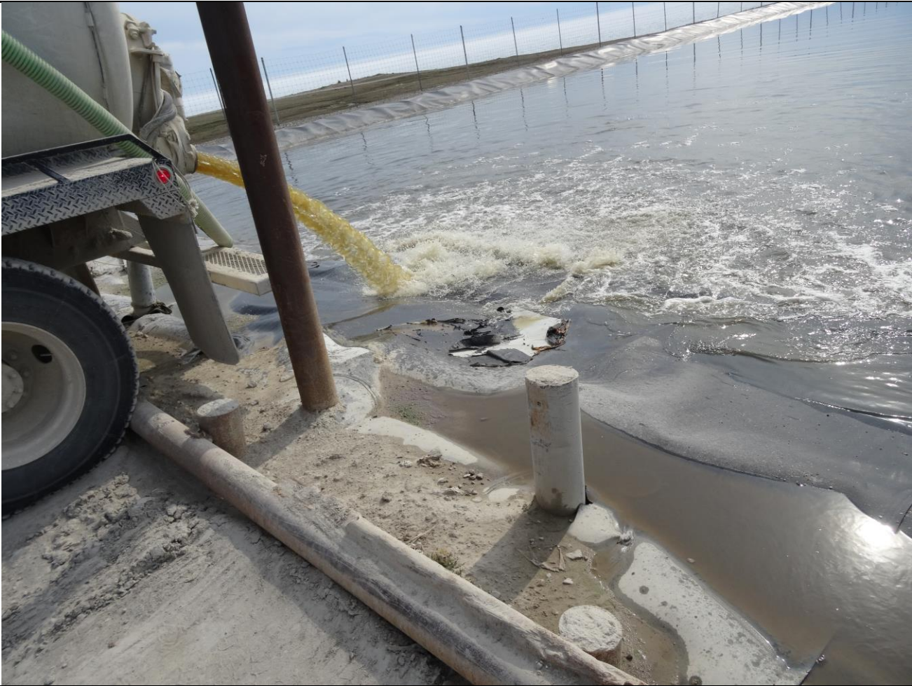
Description: Tear in Lagoon Liner requires Repair after Decant Program is complete
