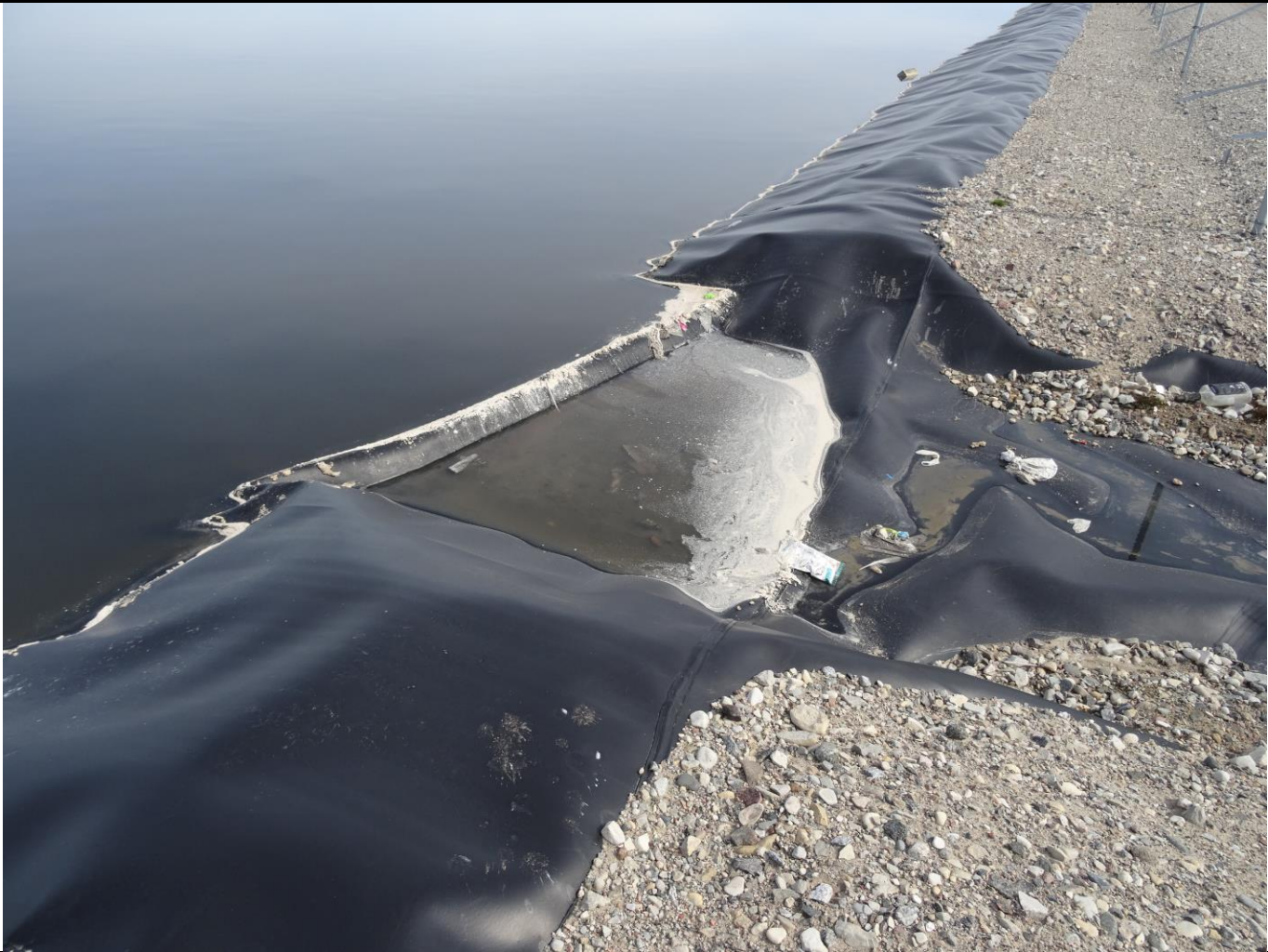
Description: No Freeboard at Emergency Runoff, Lagoon requires Decant
