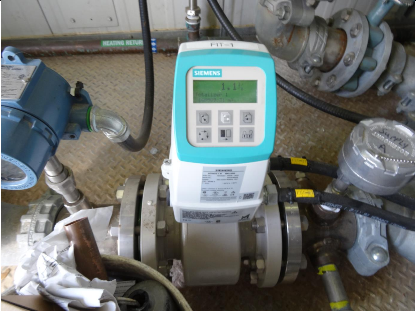
Description: Raw Water Flow Meter inside Swan Lake Pump House – Very Nice
