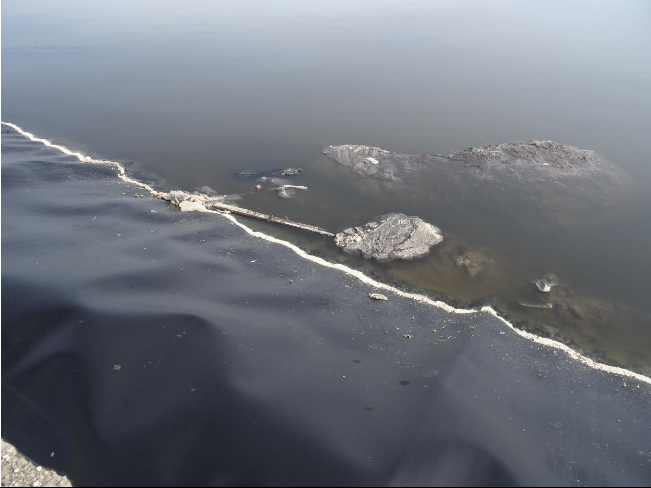
Description: Floating Debris within Sewage Lagoon requires Removal
