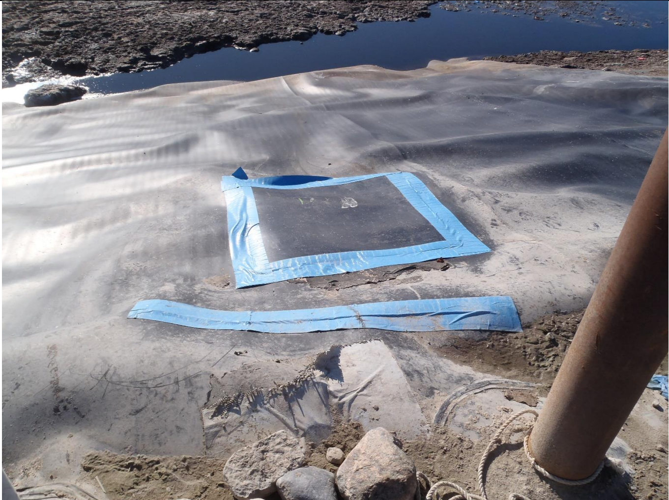
Description: Hole in Sewage Lagoon Liner AFTER REPAIR as at 2020 September 9
