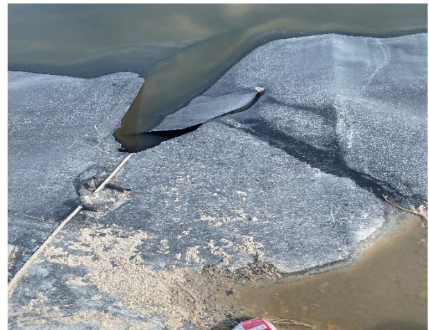
Figure 3b: Gjoa Haven Liner Tear, June 2024
