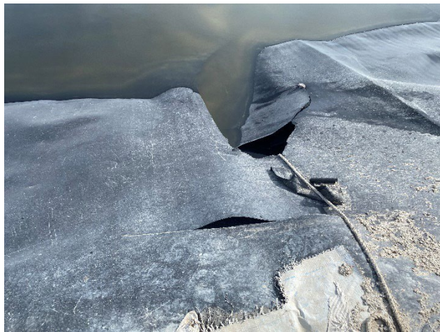
Figure 3a: Gjoa Haven Liner Tear, June 2024
