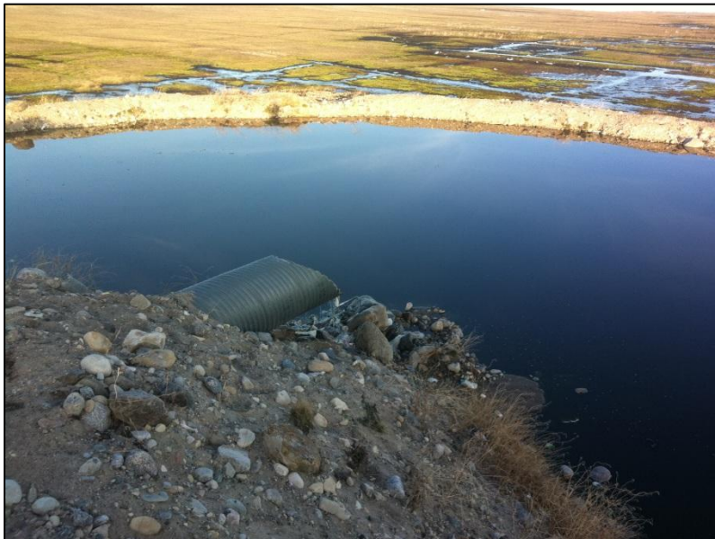
Photo 3: Sewage Treatment Pipe Outflow on Existing Lagoon
