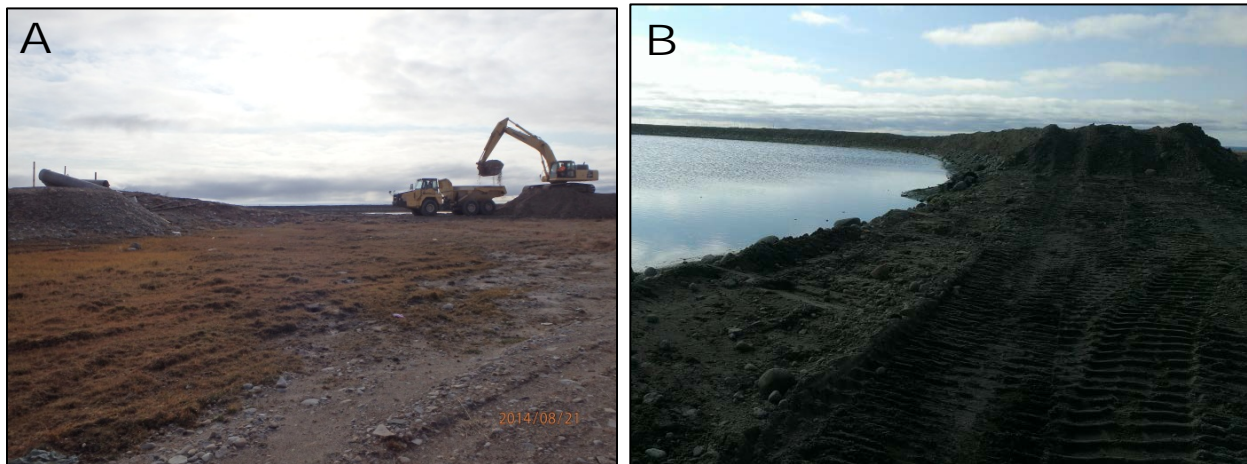
Photo 7: a – Removal of berm material at north end of site, b – Graded berm at north end of site
