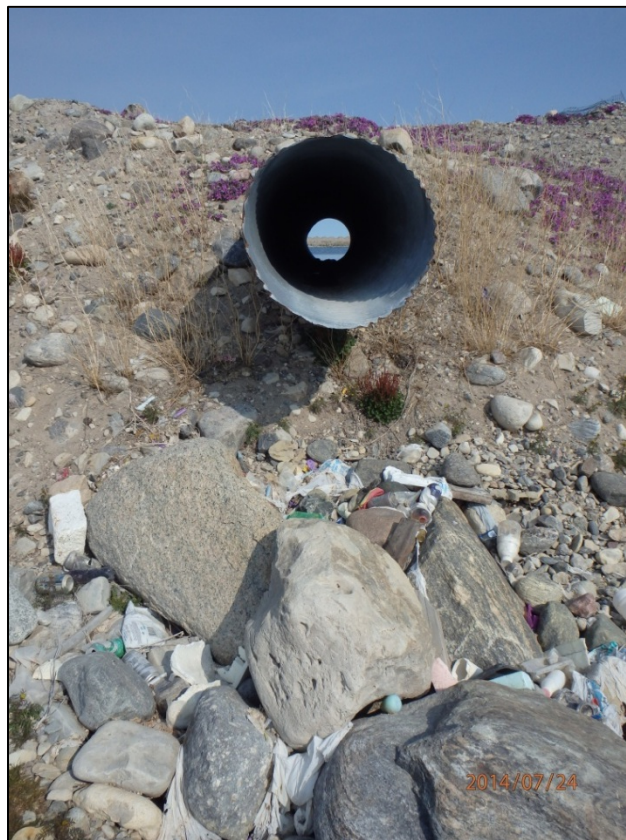
Photo 6: Outflow pipe to secondary containment berm
