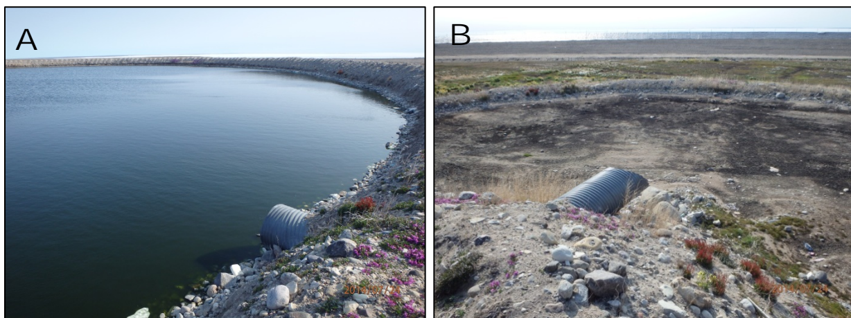
Photo 2: a – Former lagoon outflow pipe, b – Secondary containment cell
