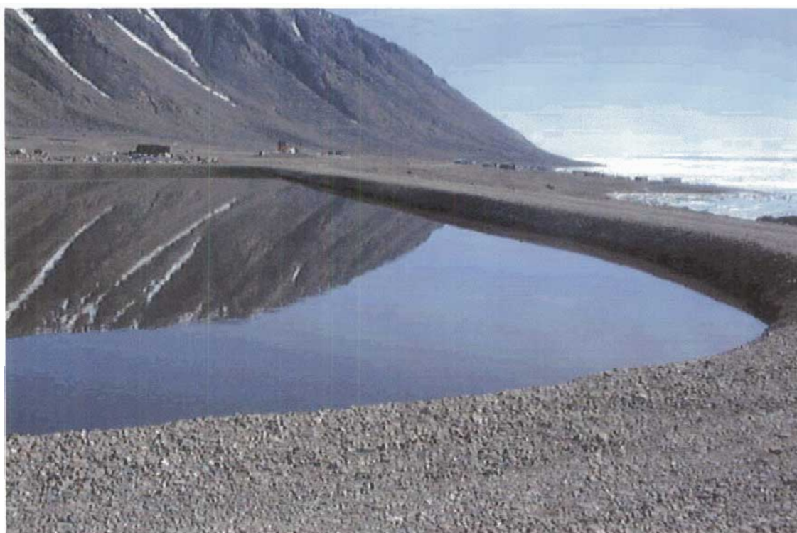
figure 2. Limited freeboard at the sewage disposal facility; 2001/07/20.
