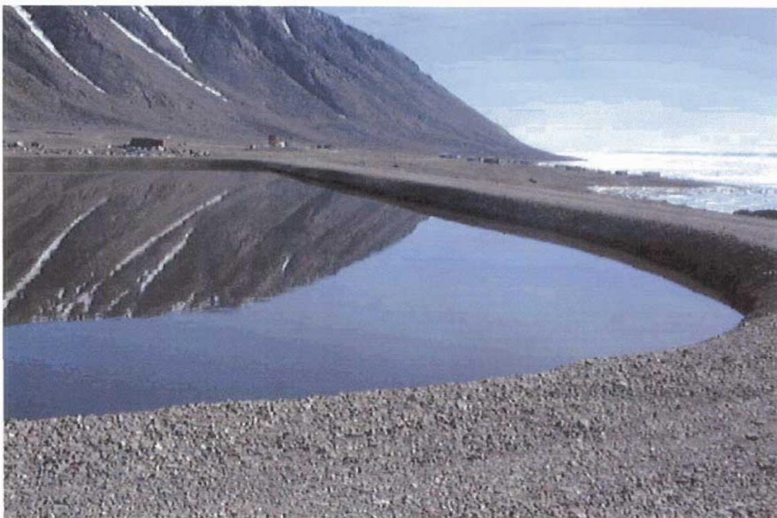
figure 2. Limited freeboard at the sewage disposal facility; 2001/07/20.
