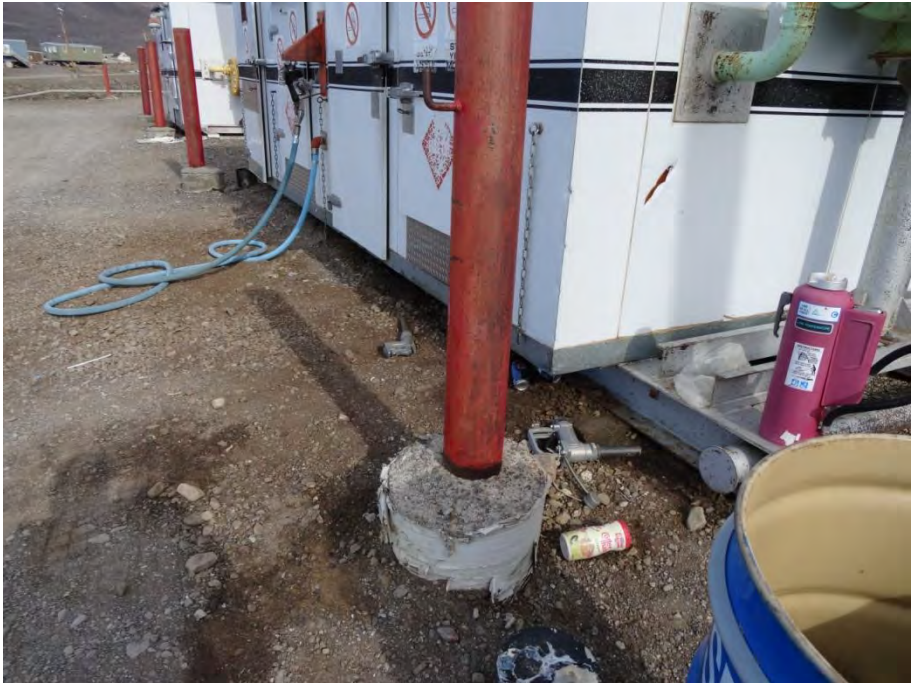
Figure 6 Fuel staining and hydrocarbon contaminated soils at site of spill
