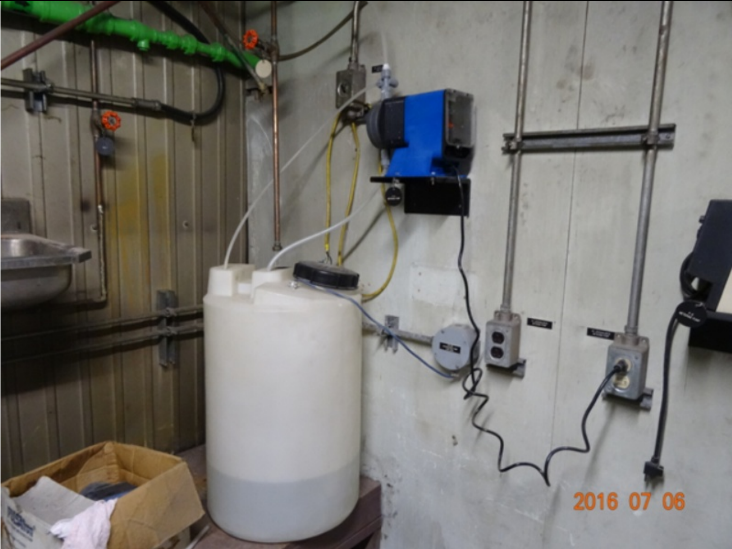
Figure 17Water treatment system at garage. Noted corrosion/oxidation of metals and fittings in room.
