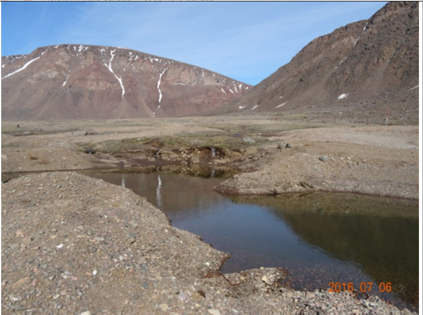
Figure 1 Raw water intake. Pond has been expanded to create a new cell
