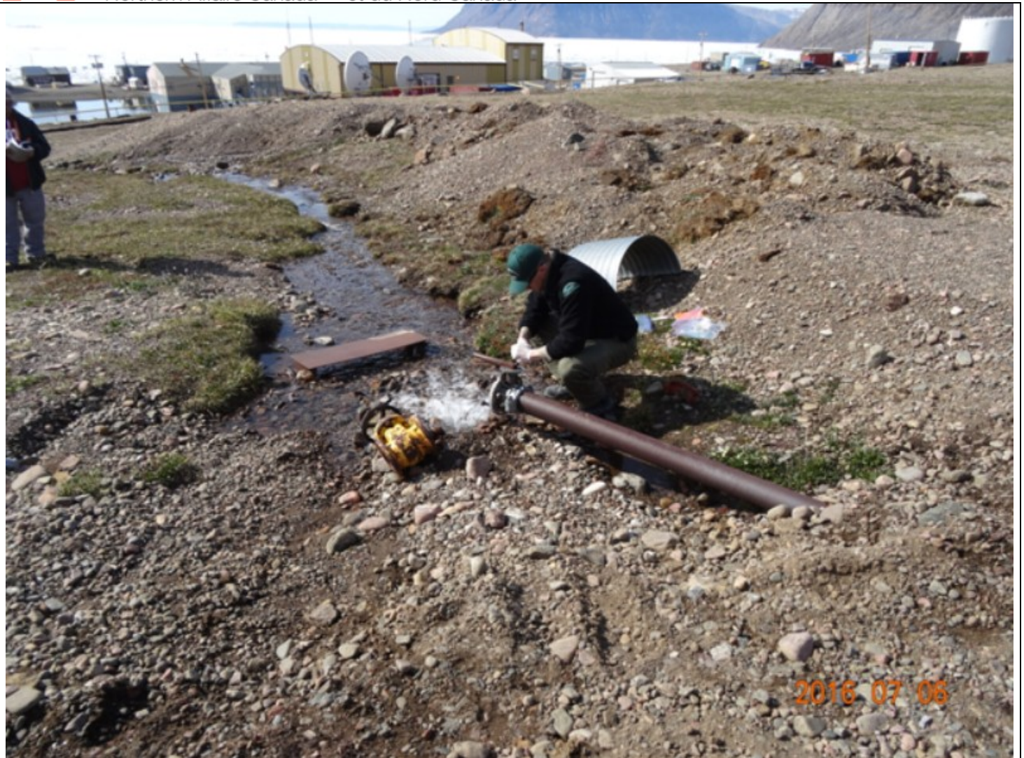
Figure 3 Pipe to fill tanks. tanks just recently filled so pipe is disconnected . Samples collected
