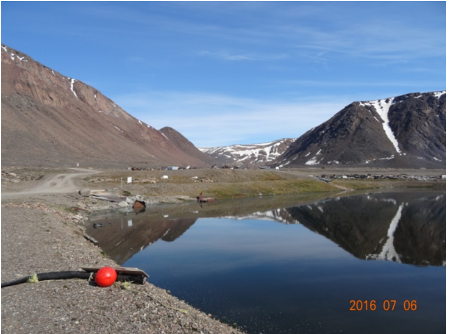
Figure 12 Decant hose on top of berm wall
